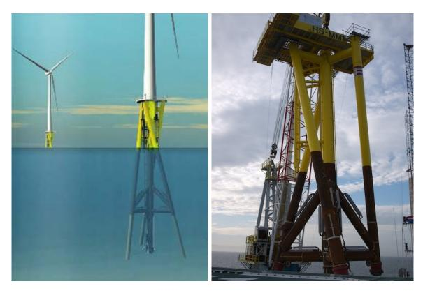
Figure 2. Inward Battered Guide Structure (IBGS) or "twisted jacket" foundation support structure for wind turbines. Left: Keystone Engineering. Right: National Renewable Energy Laboratory
