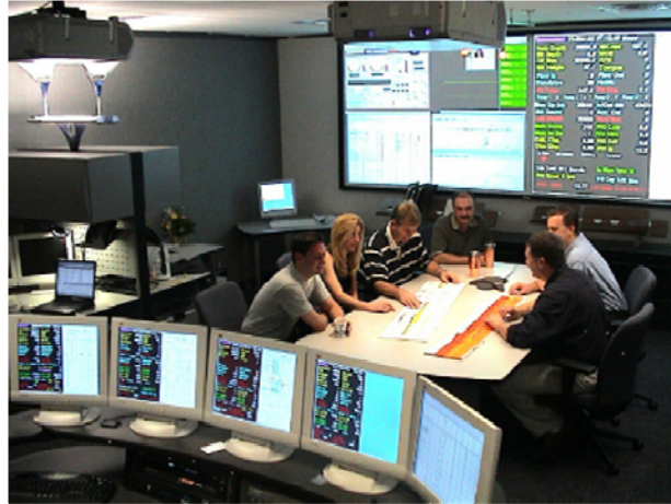
FIGURE 2-2 REAL TIME OPERATIONS CENTER
