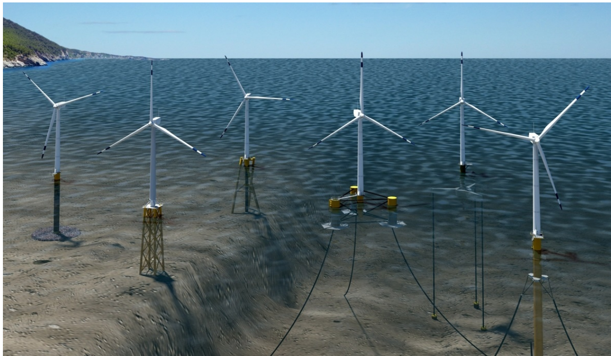
Figure 1: Offshore wind foundation types
