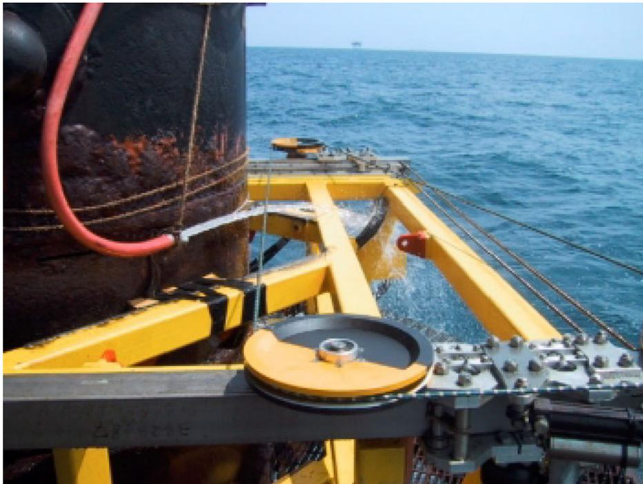
Figure 6.4. Diamond Wire Cutting System Applied to a 72-inch Deck Leg on the Surface (Courtesy of CUT USA, Inc.).
