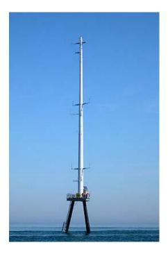
Figure 3-1 Example of Monopole Mast Meteorological Tower with a Tripod Foundation
