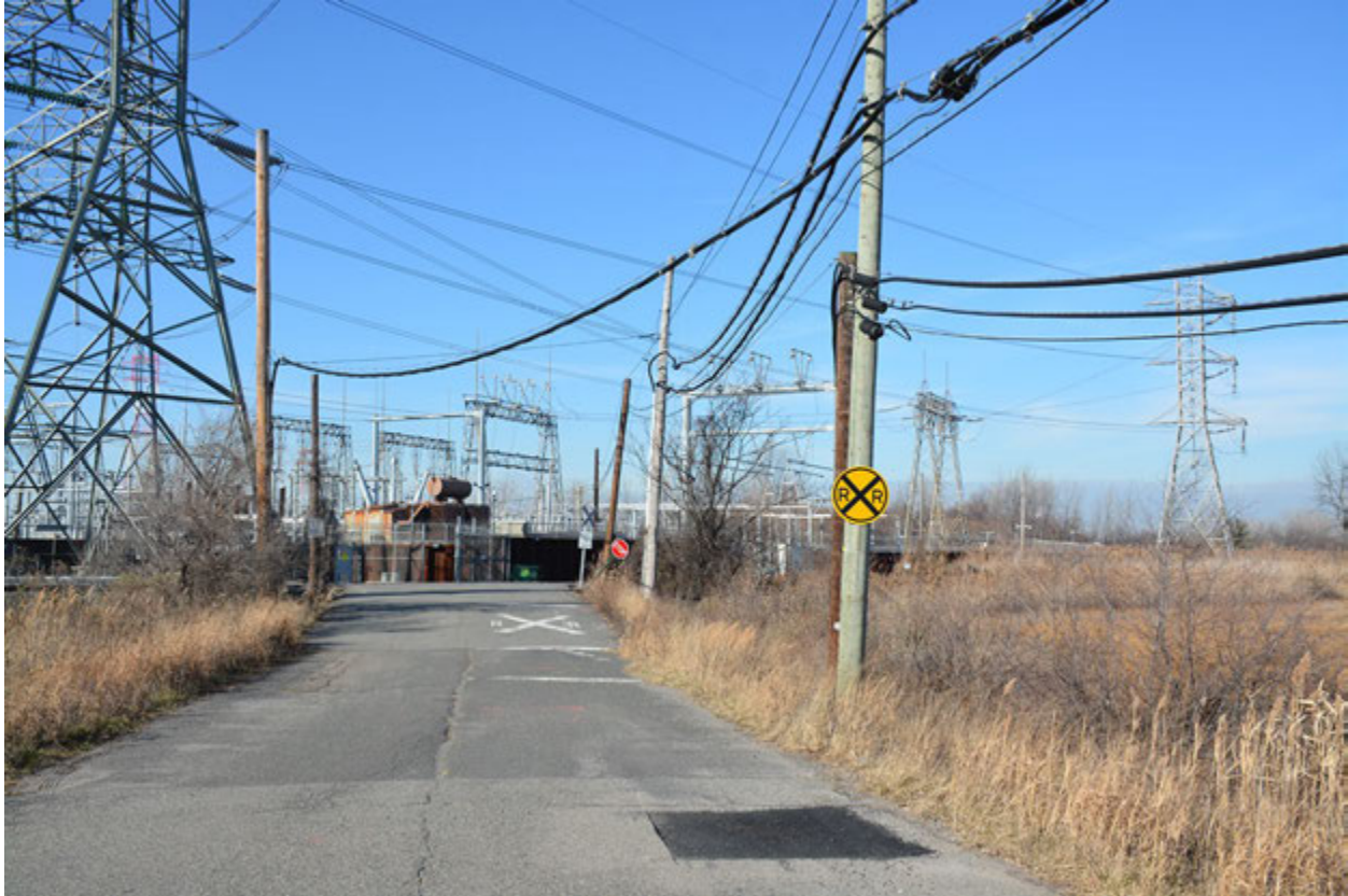
Inset 9.8-19. Existing View of the River Road Site from KOP 19
