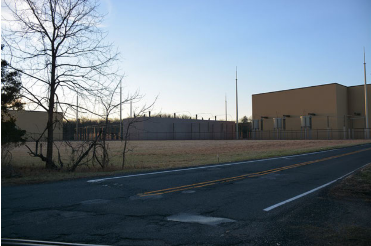
Inset 9.8-2. Photosimulation of the Lanes Pond Road Substation/Converter Station from KOP 46
