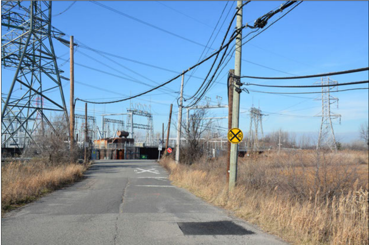
Inset 9.6-9. Representative KOP of the River Road Site
