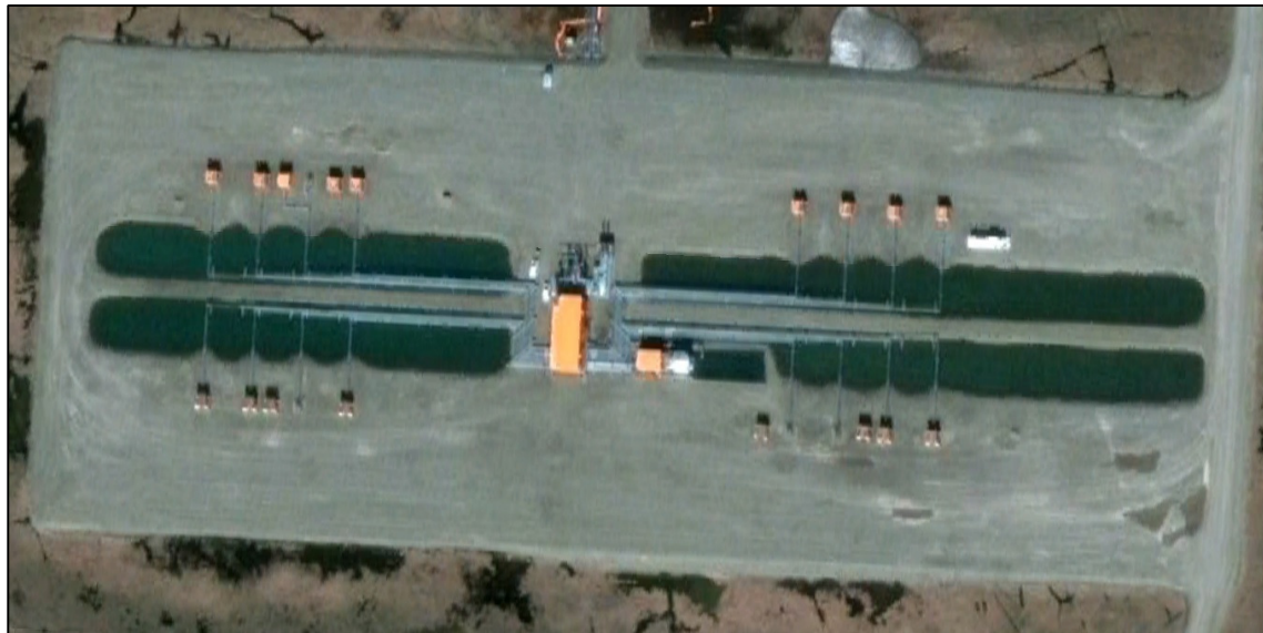
Figure III-4. Typical North Slope Well Pad
