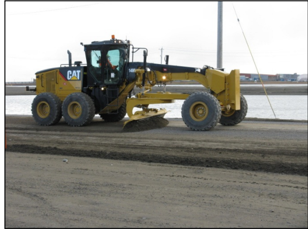
Figure III-15. Grader Leveling Barrow Unpaved Road
