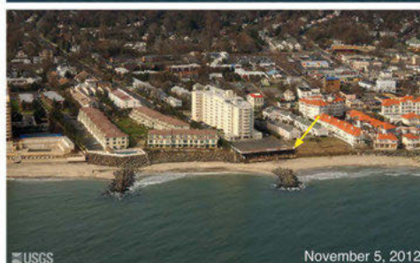
Beach erosion in Long Branch, NJ. Photos by U.S. Geological Survey.
