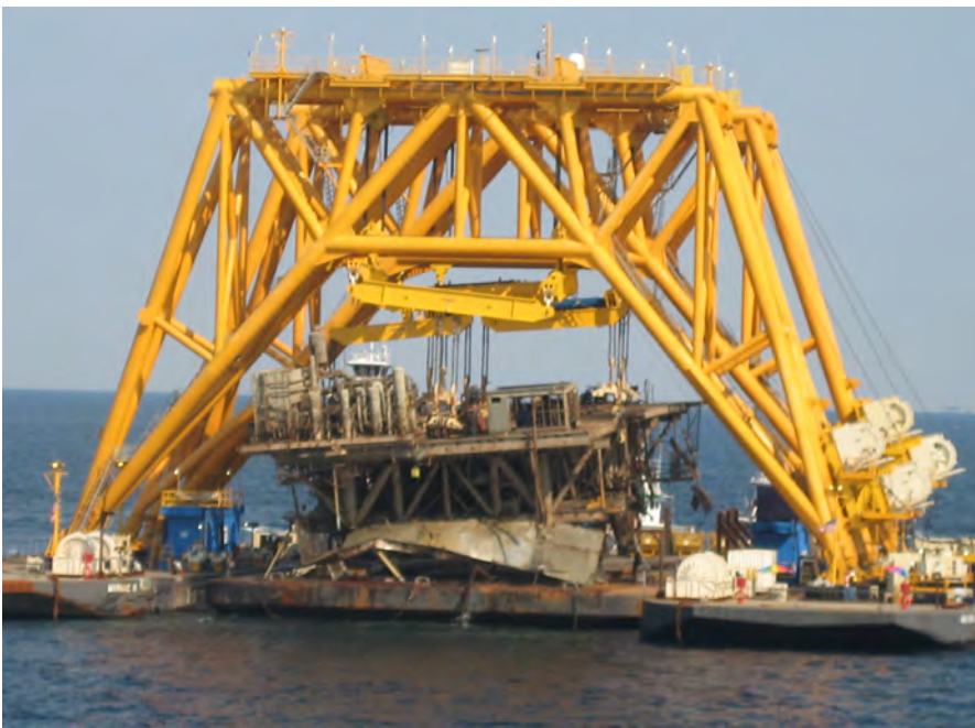
Main Pass 306 E, a platform in the Gulf of Mexico, was toppled and destroyed during Hurricane Ivan in September 2004. Here, a specially-rigged lift vessel (yellow structure) is removing the toppled platform's deck, which it retrieved from the seafloor.
