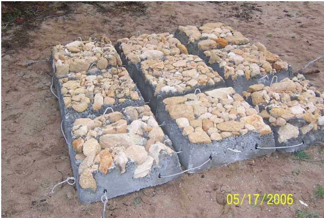
Figure 6-5. Articulated Concrete Mattress
