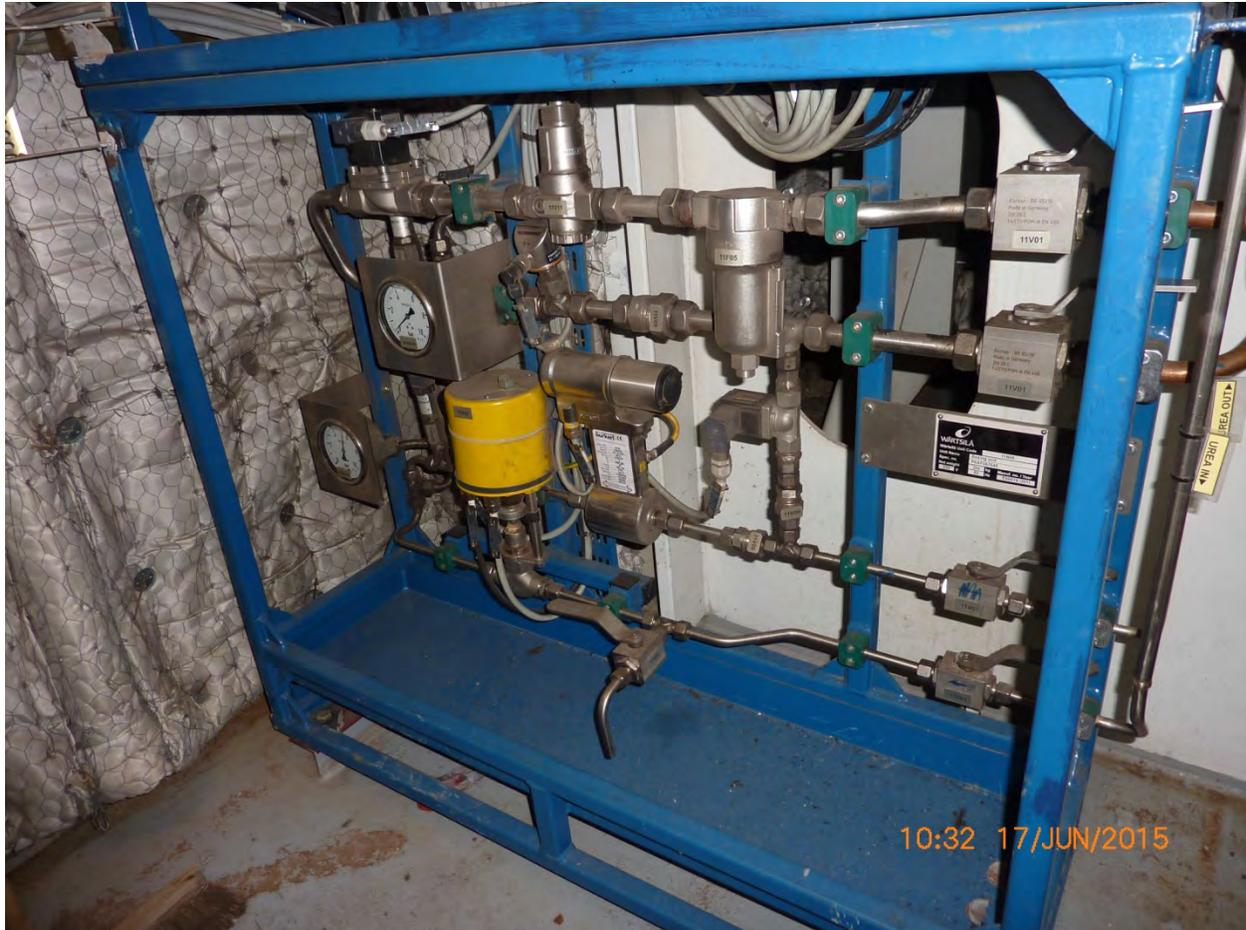
Nordica 15 – Main Engine No. 1 – SCR control valves
