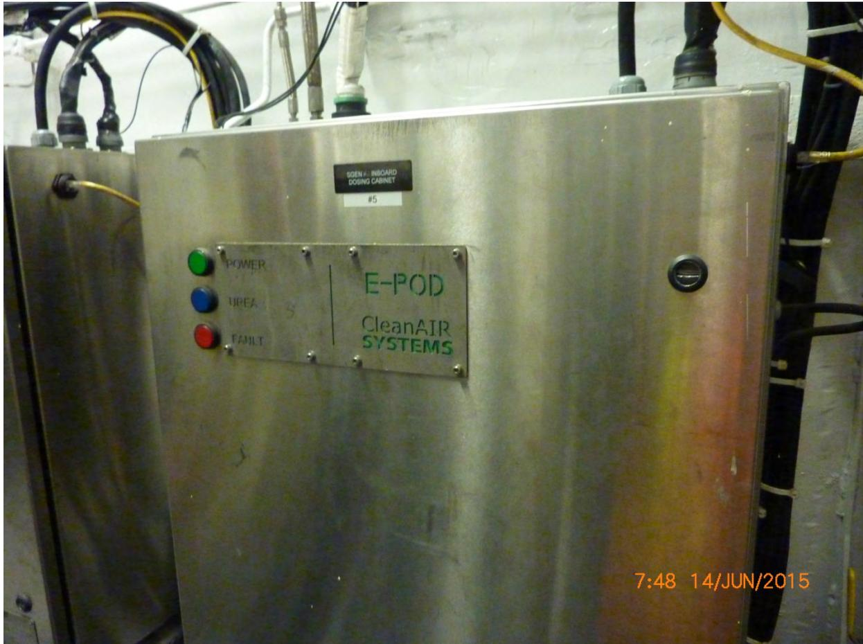
Aiviq 10 – Generator Engine No. 4 – SCR urea control panel
