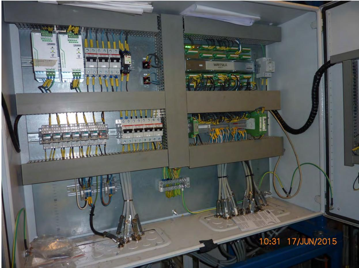
Nordica 17 – Main Engine No. 4 – SCR control panel (inside)
