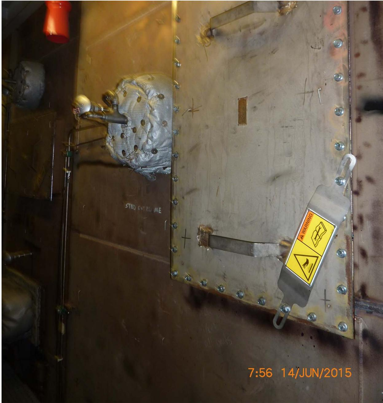
Aiviq 1 – Main Engine No. 4 – Diesel oxidation catalyst housing and urea entry port
