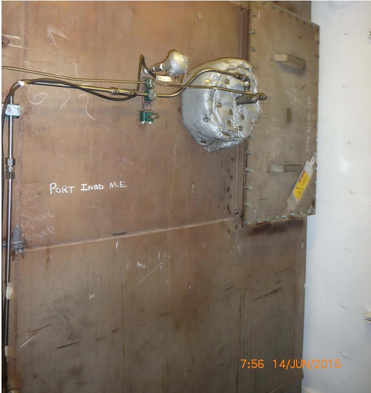
Aiviq 3 – Generator Engine No. 4 – Catalyzed diesel particulate filter housing
