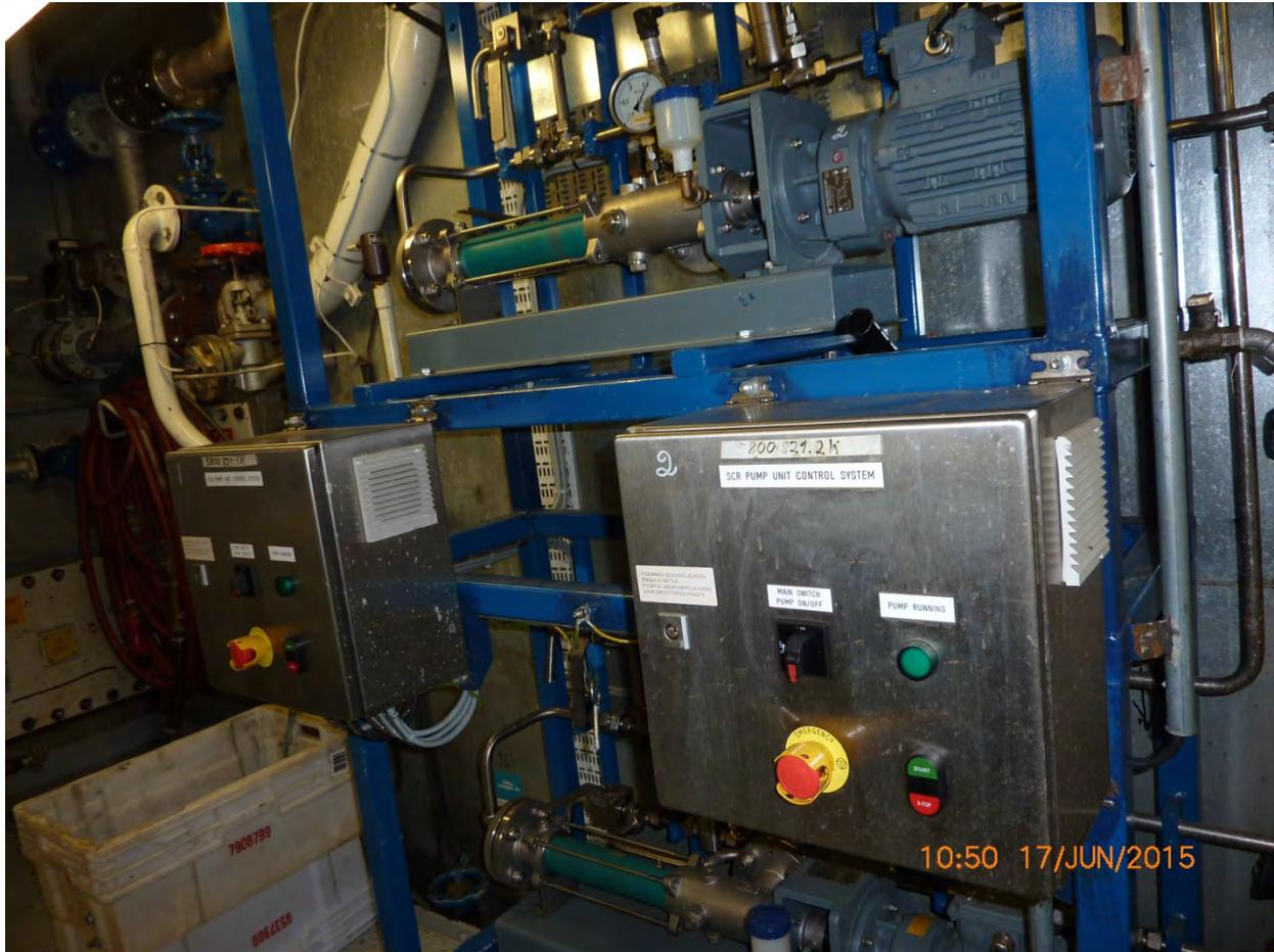
Nordica 3 – SCR Pump Control Panel No. 2 and Urea Pump
