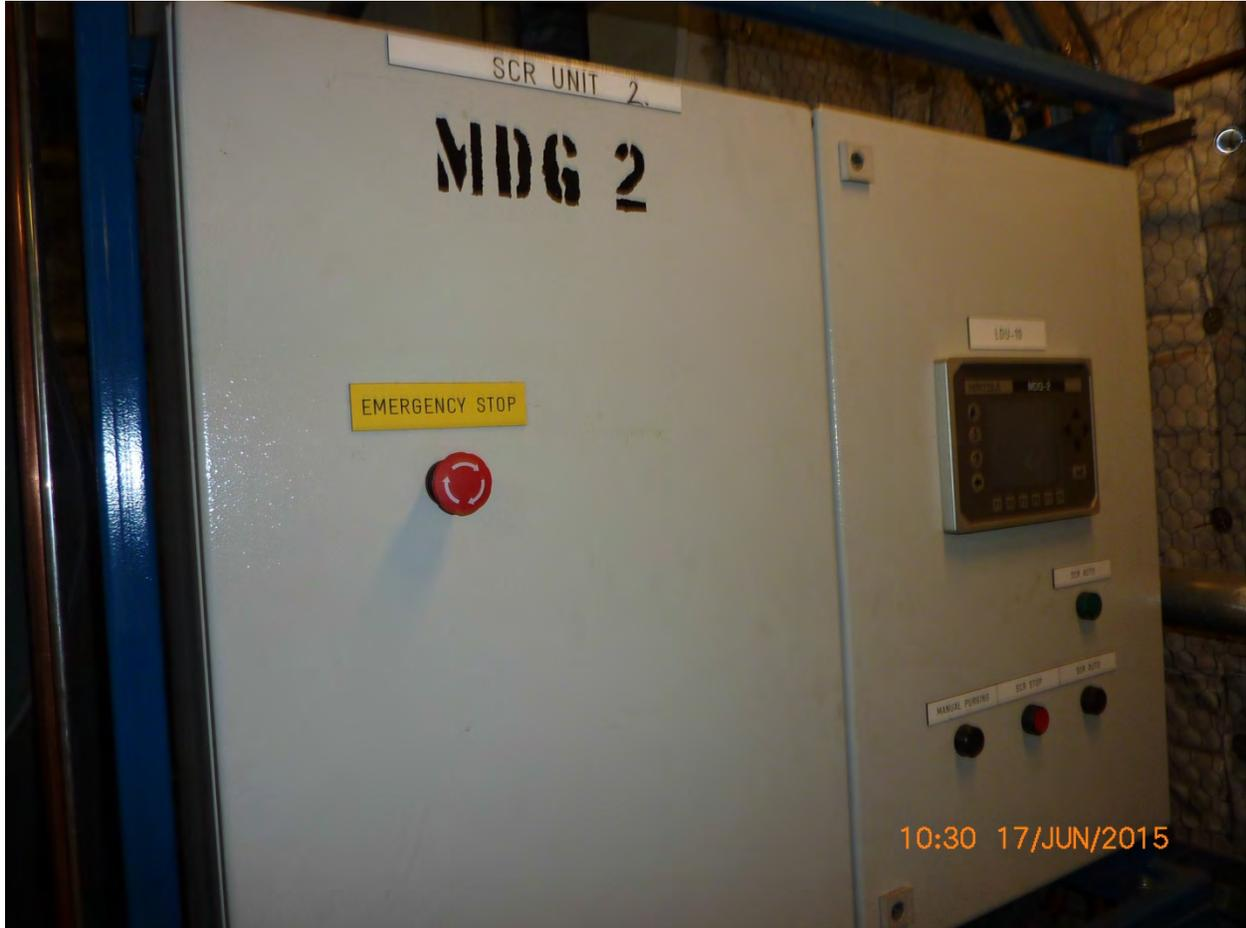
Nordica 21 – Main Engine No. 2 – SCR control panel
