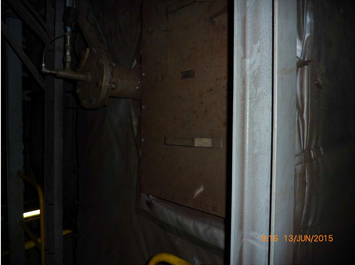
Noble Discoverer 19 – Main Generator Engine No. 5 -- Catalyzed diesel particulate filter housing
