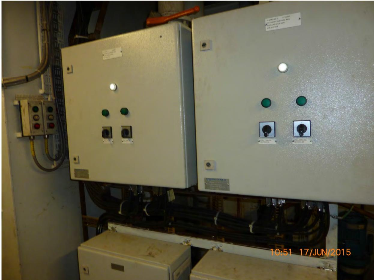
Nordica 2 – SCR Tank Heater Panel
