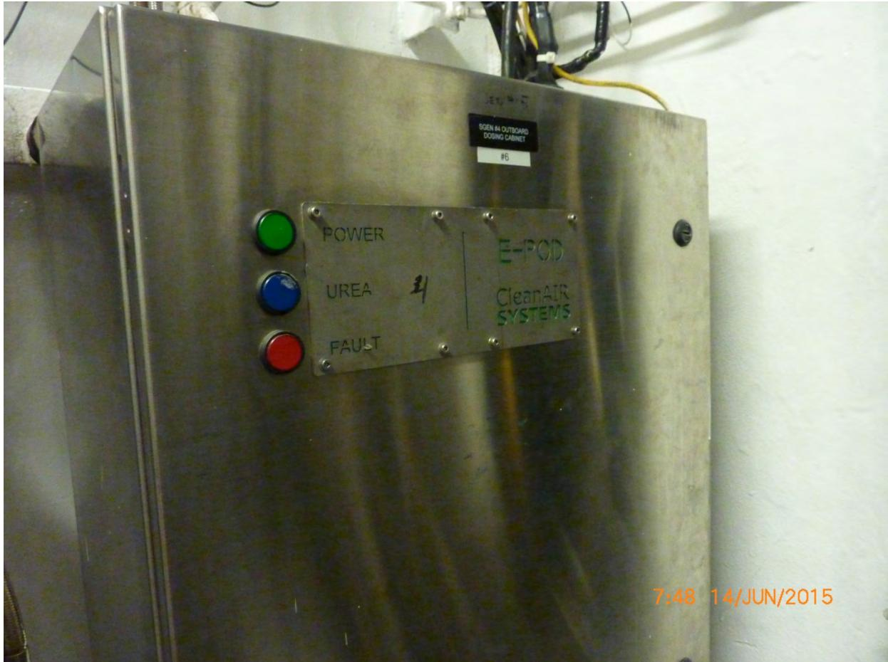
Aiviq 9 – Generator Engine No. 5 – SCR urea control panel
