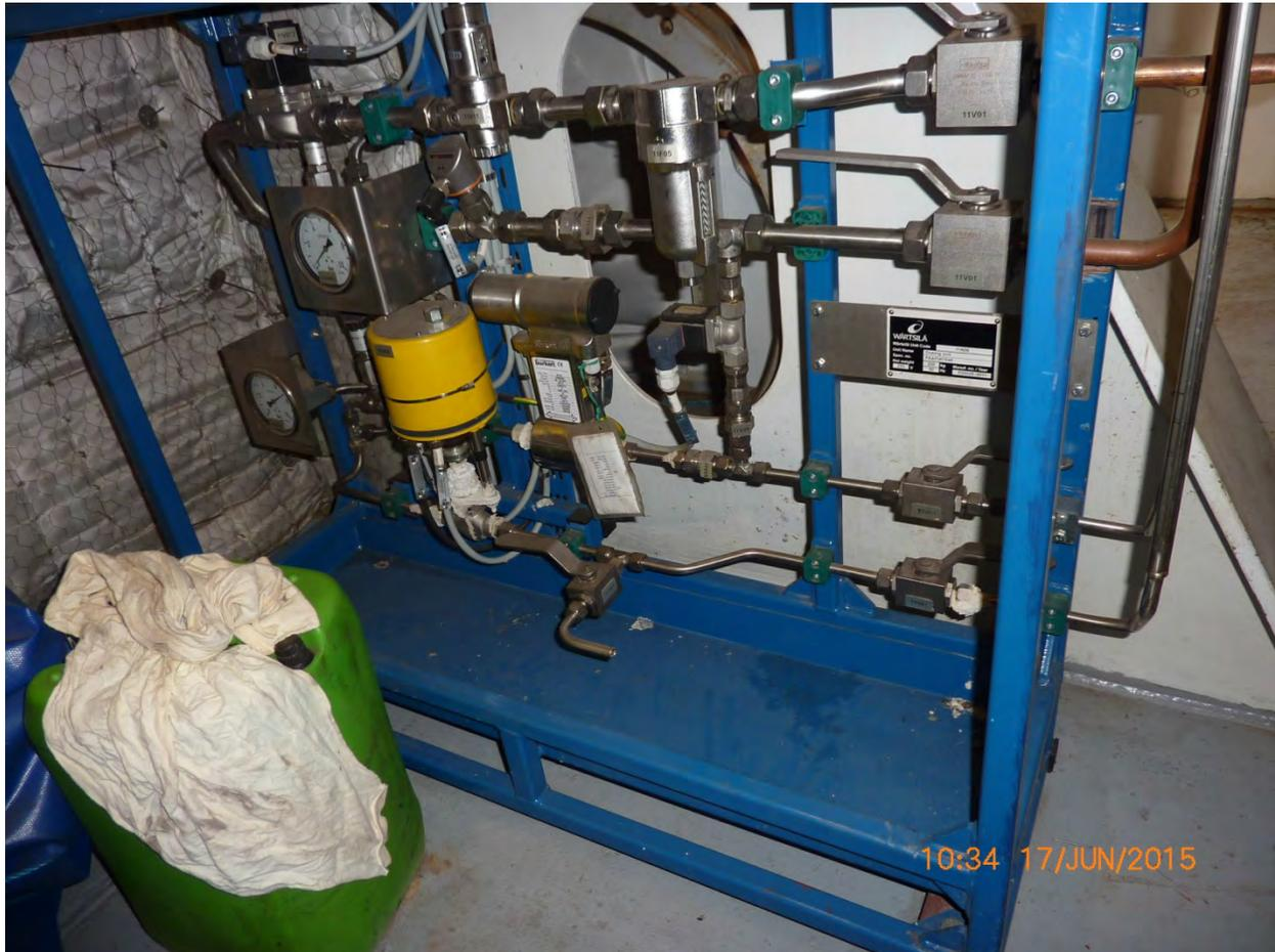
Nordica 13 – Main Engine No. 3 – SCR control valves
