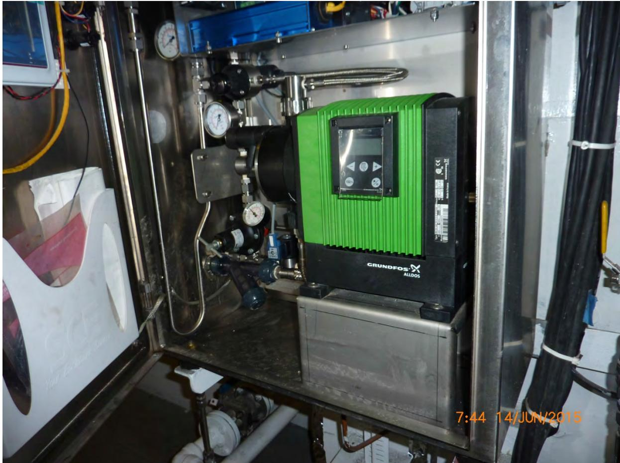
Aiviq 16 – Main Engine No. 1 – SCR urea control panel (inside)
