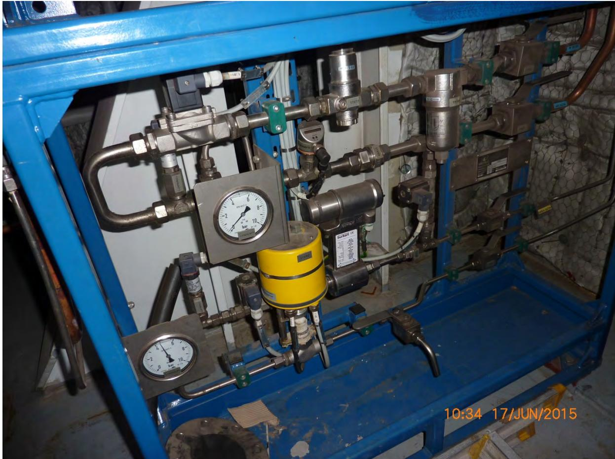
Nordica 14 – Main Engine No. 2 – SCR control valves
