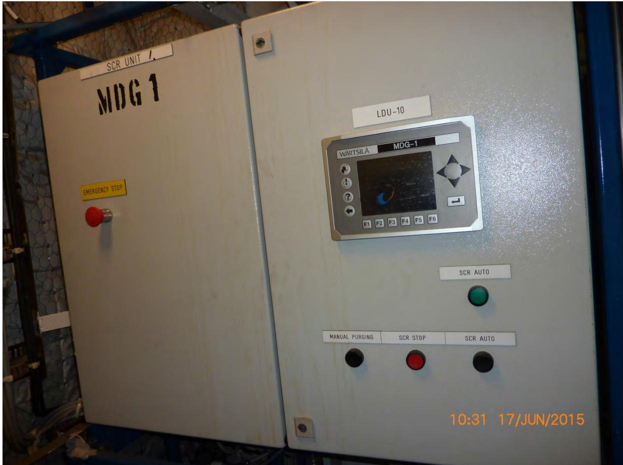
Nordica 18 – Main Engine No. 1 – SCR control panel
