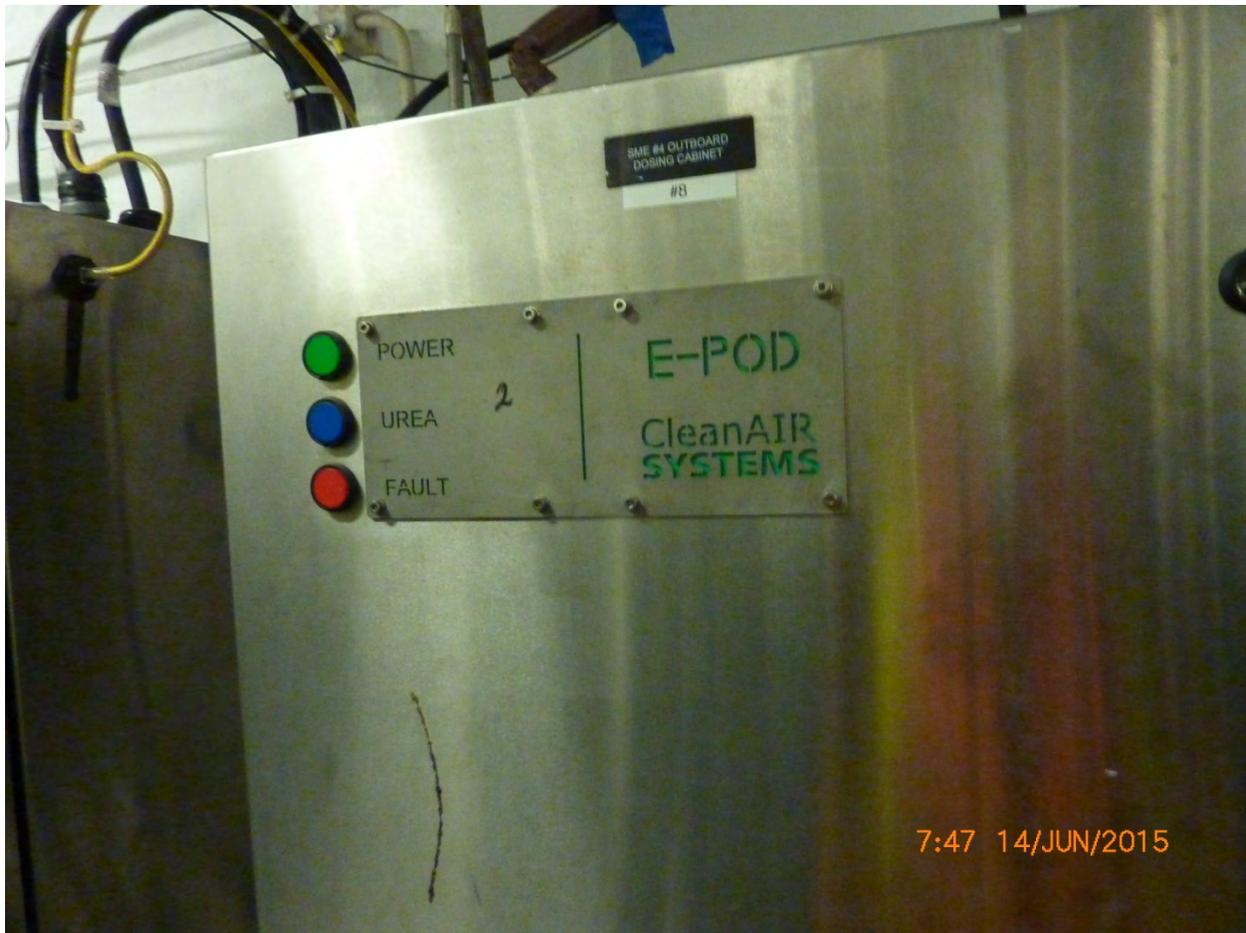
Aiviq 13 – Main Engine No. 4 – SCR urea control panel
