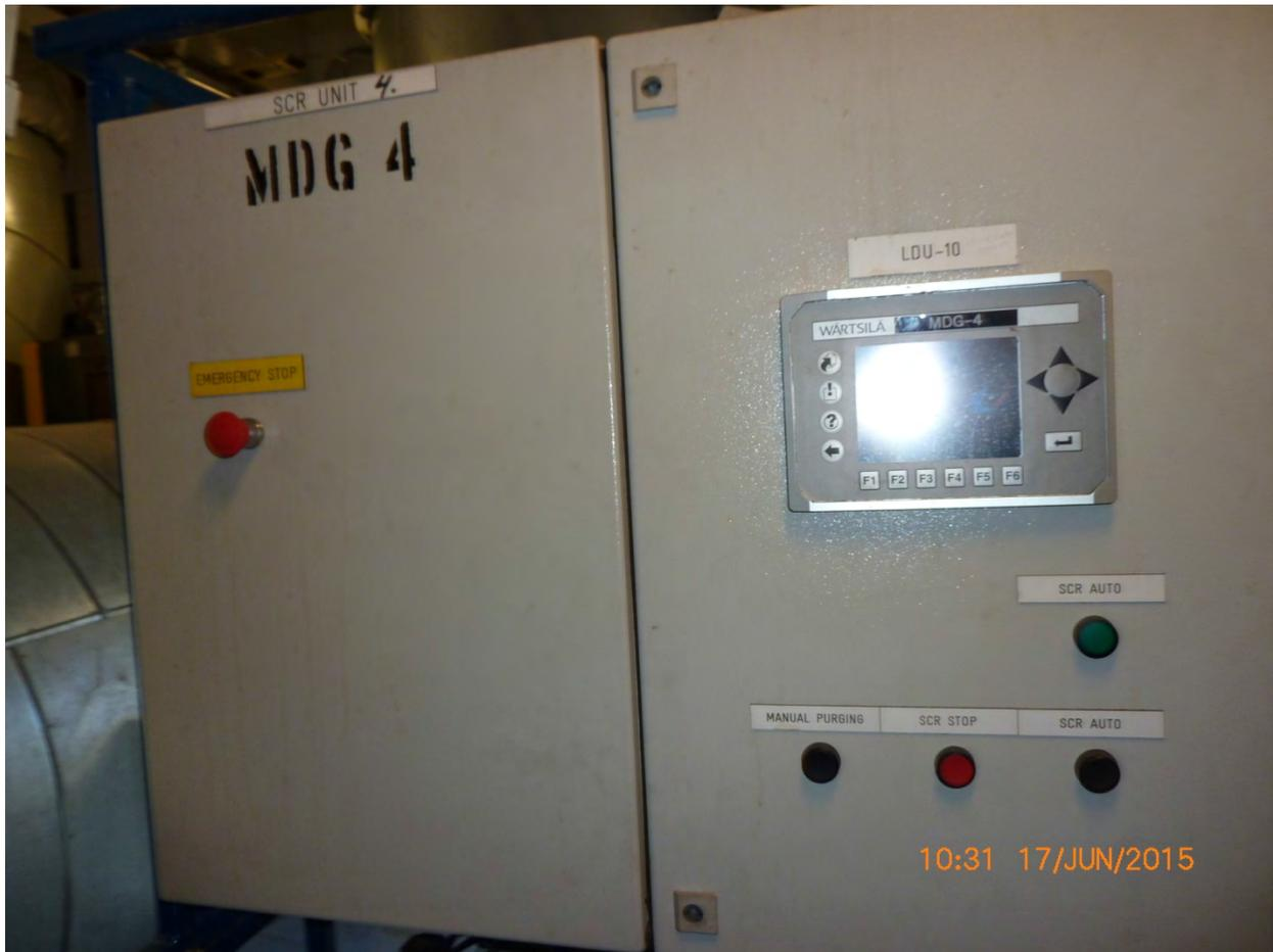
Nordica 19 – Main Engine No. 4 – SCR control panel
