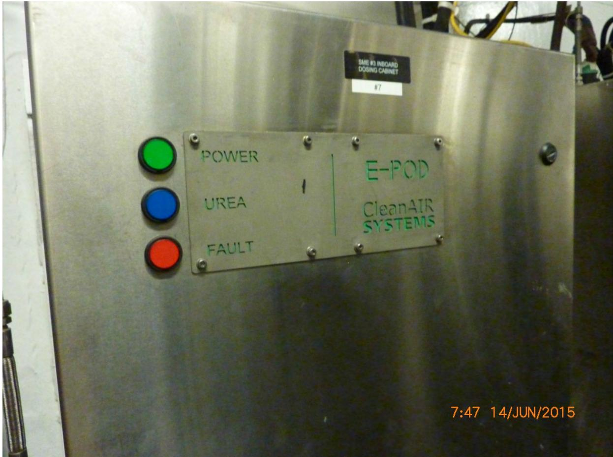
Aiviq 14 – Main Engine No. 3 – SCR urea control panel
