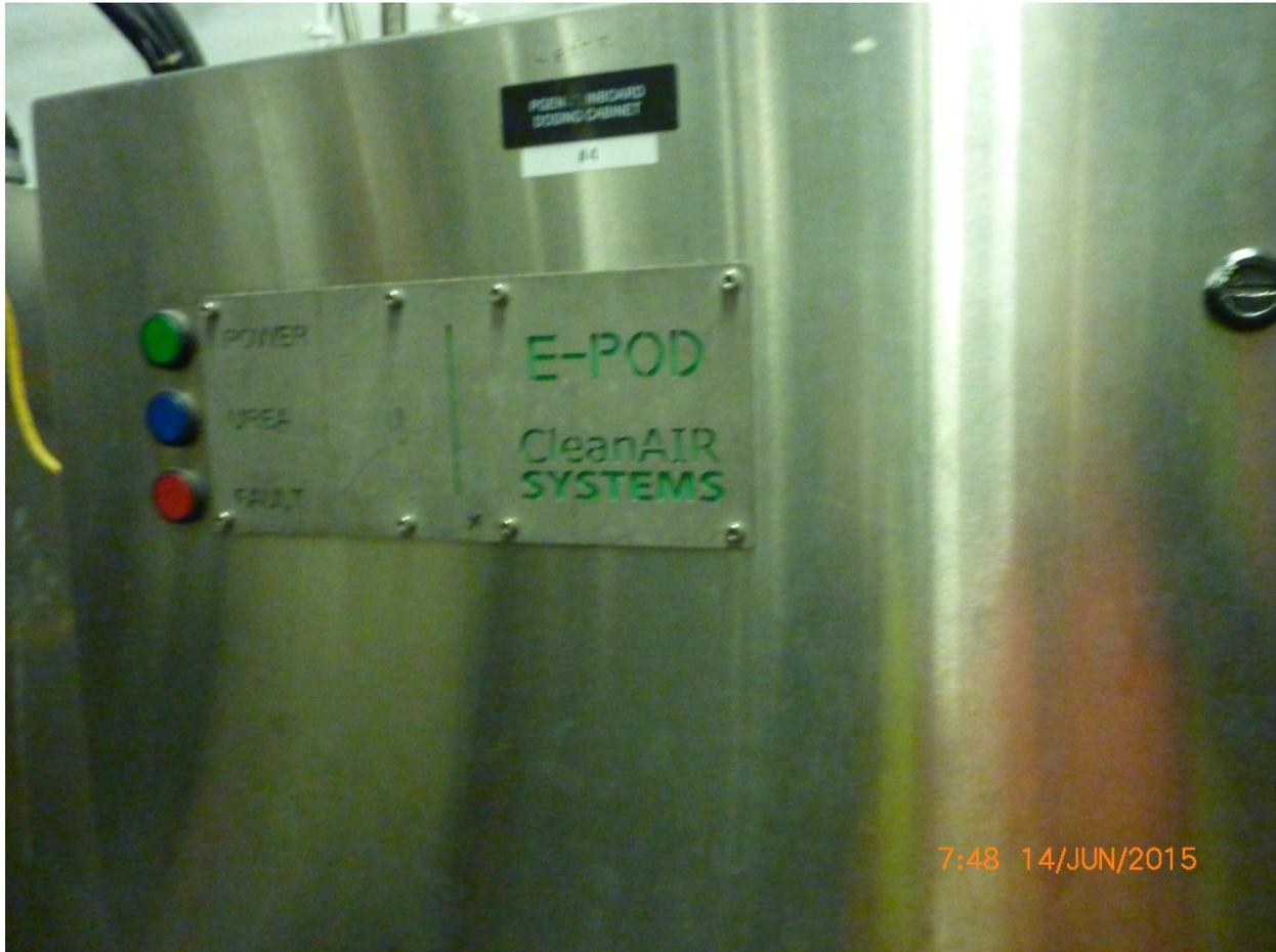
Aiviq 11 – Generator Engine No. 3 – SCR urea control panel
