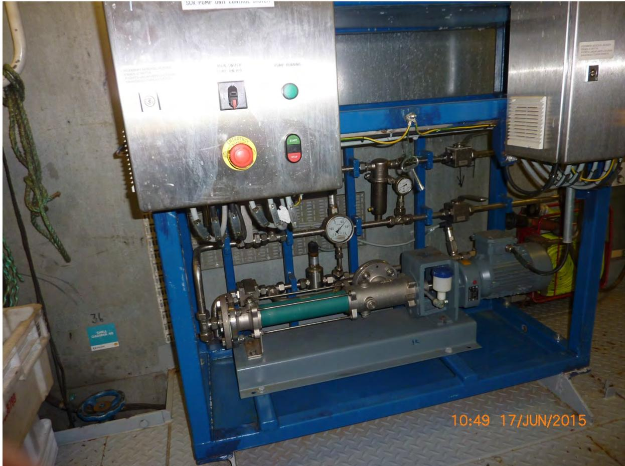
Nordica 4 – SCR Pump Control Panel No. 1 and Urea Pump
