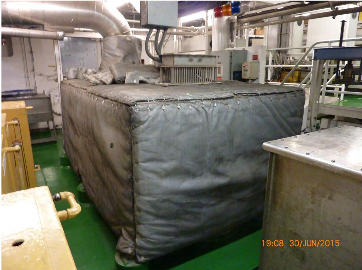
Nanuq 3 – Forward Generator Engine -- Catalyzed Diesel Particulate Filter Housing
