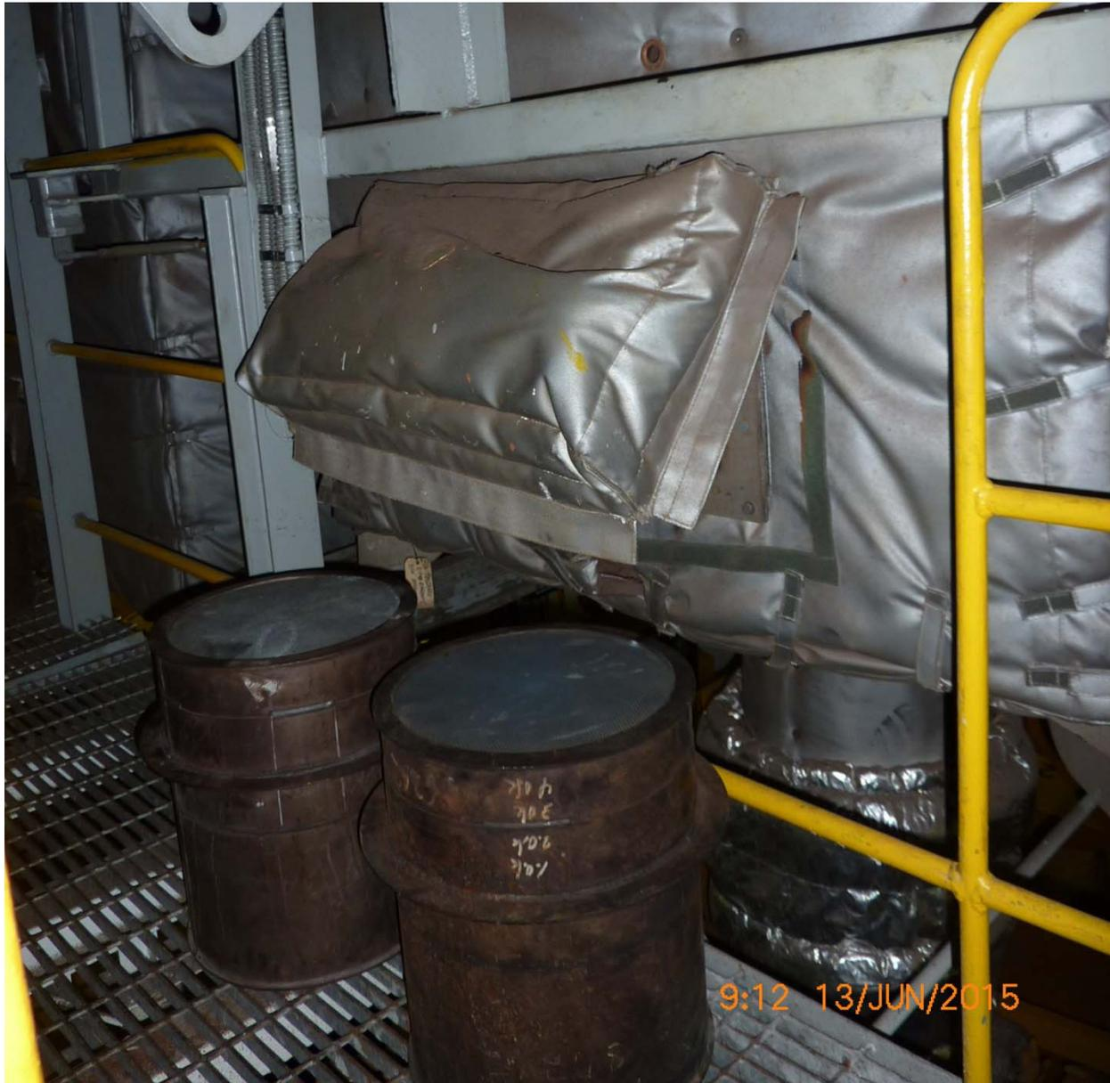
Noble Discoverer 22 – Main Generator Engine No. 2-- Catalyzed diesel particulate filter housing with filters
