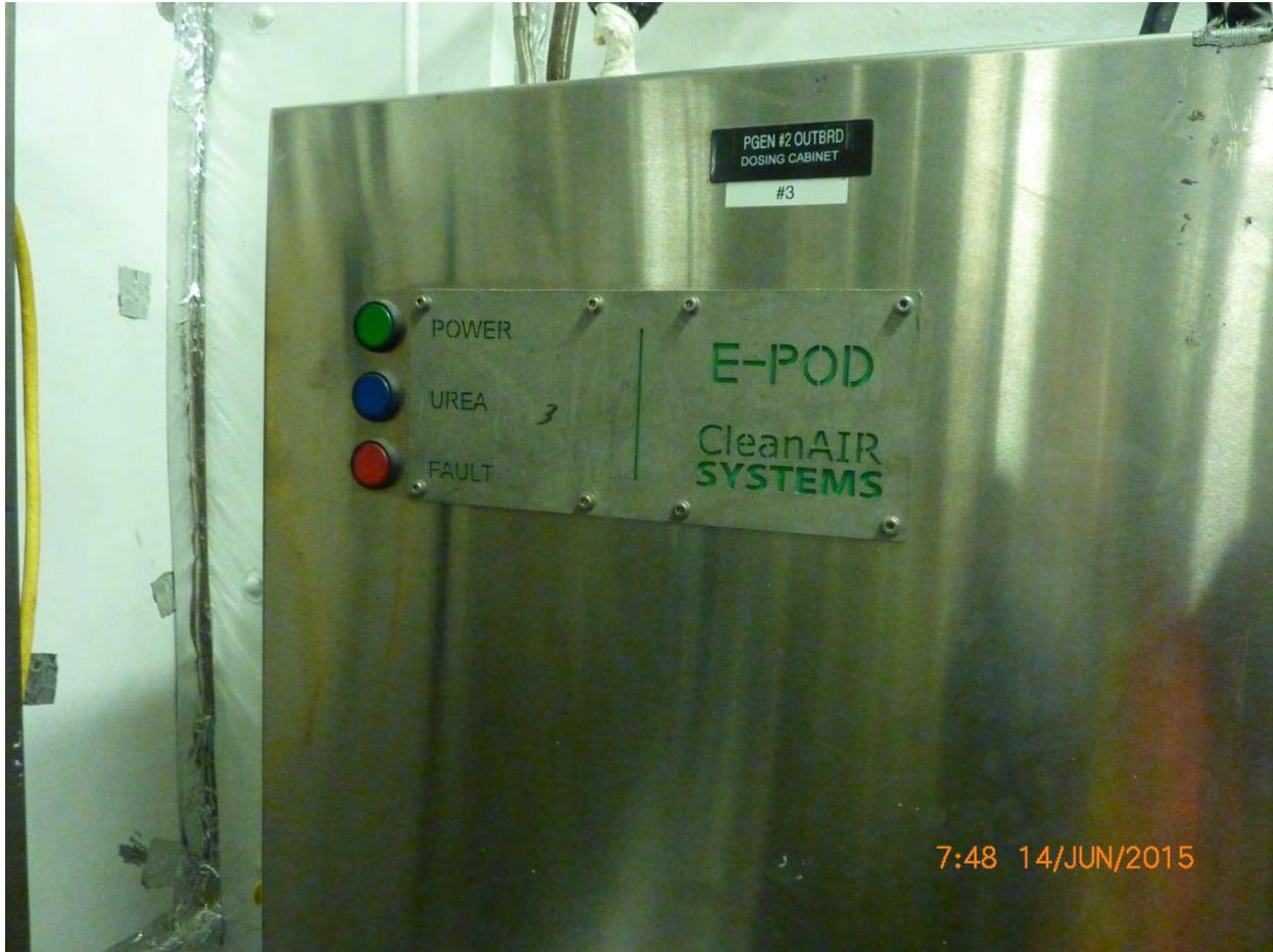
Aiviq 12 – Generator Engine No. 2 – SCR urea control panel
