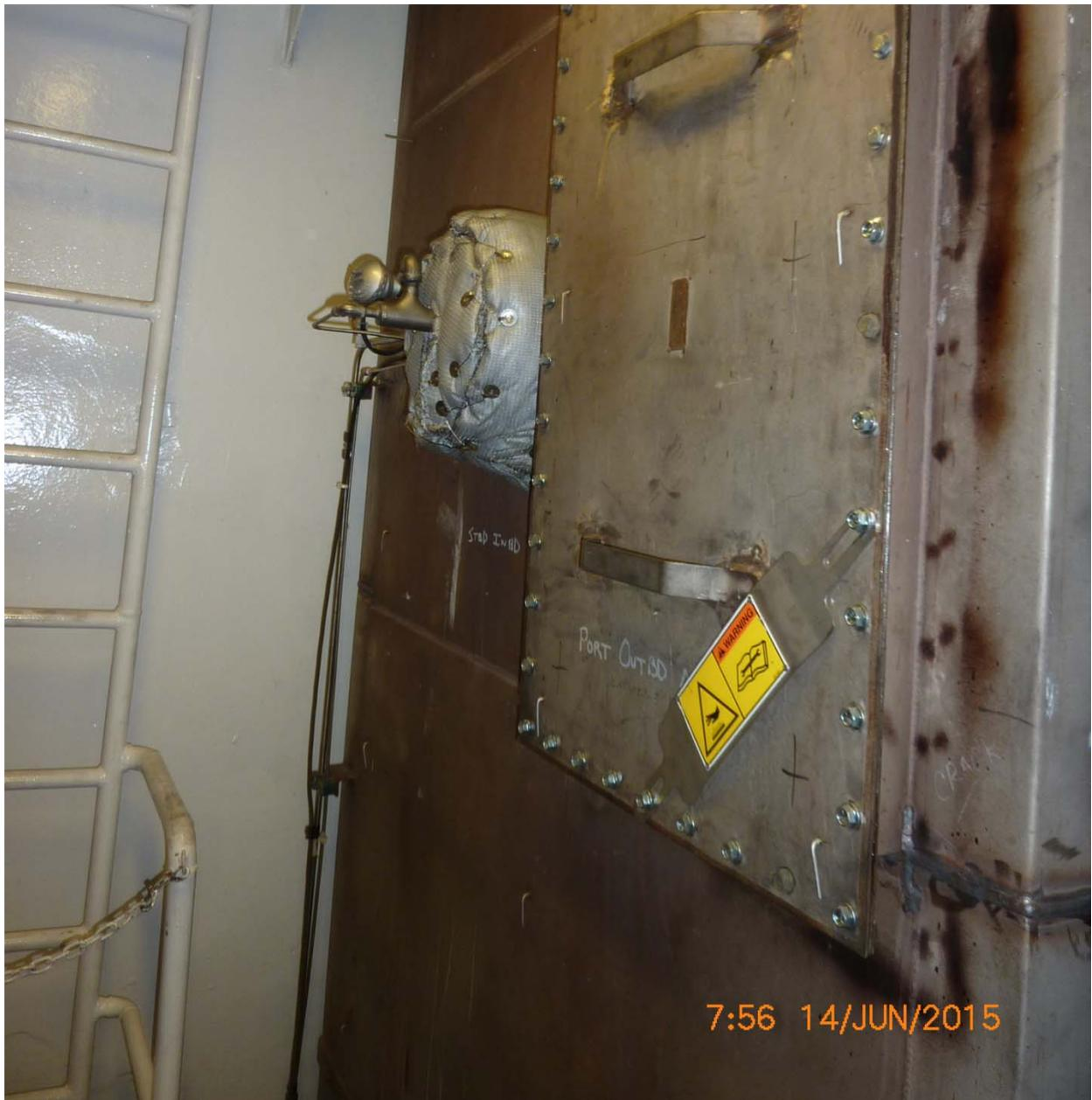
Aiviq 2– Main Engine No. 3 – Diesel oxidation catalyst housing and urea entry port
