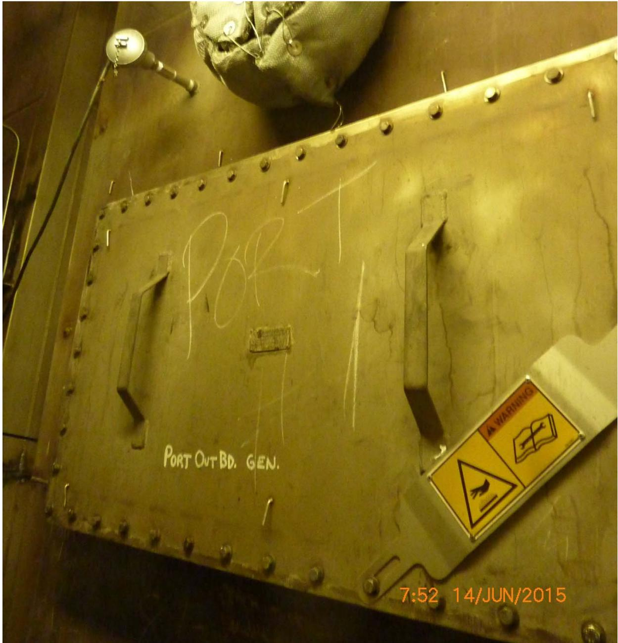
Aiviq 8 – Generator Engine No. 2 – Catalyzed diesel particulate filter housing and urea entry port
