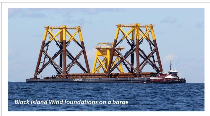
*Block Island Wind foundations on a barge*
