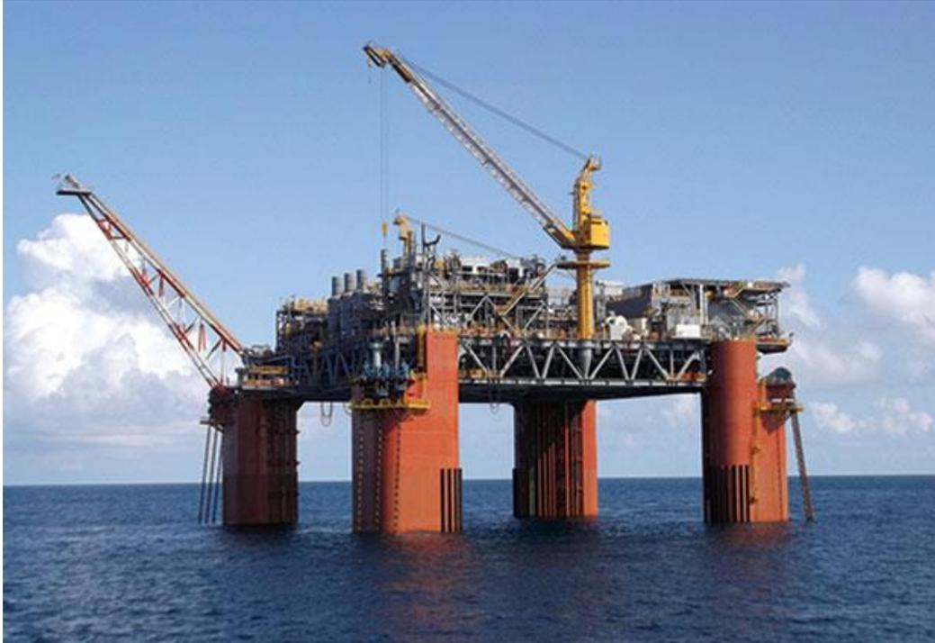
Figure S.1. Delta House semisubmersible
