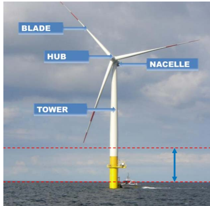
Figure 3: Anatomy of a wind turbine.
