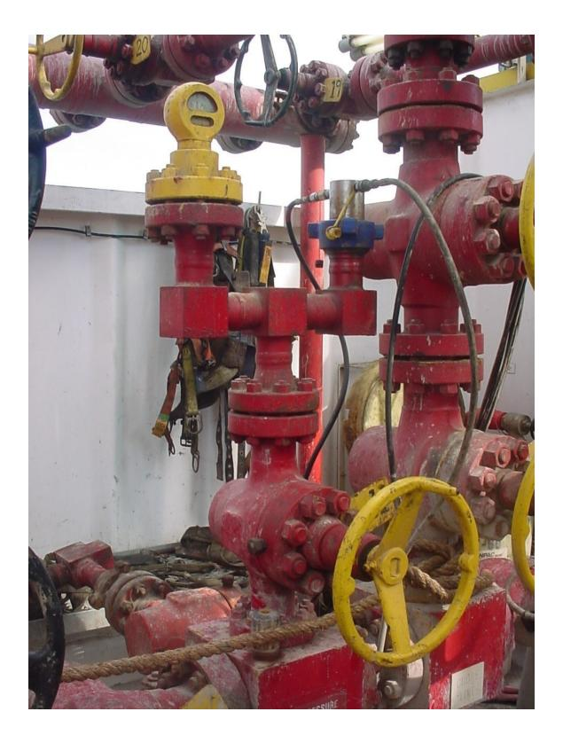
Connections for gauges on choke manifold.
