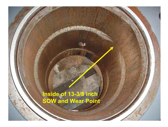
Worn and damaged 13 3/8 inch SOW, inside details.
