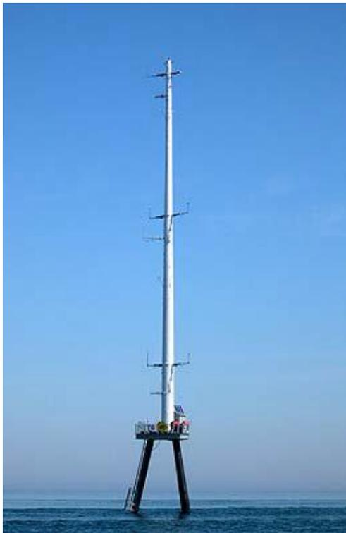
**Figure 3-5. Example of Monopole-mast Meteorological Tower**
