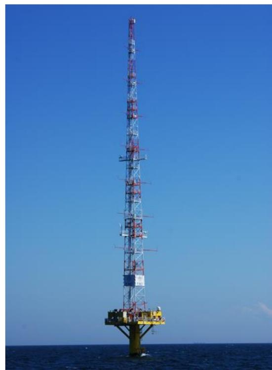
**Figure 3-6. Photograph of a Lattice-mast Meteorological Tower with a Monopile Foundation**
