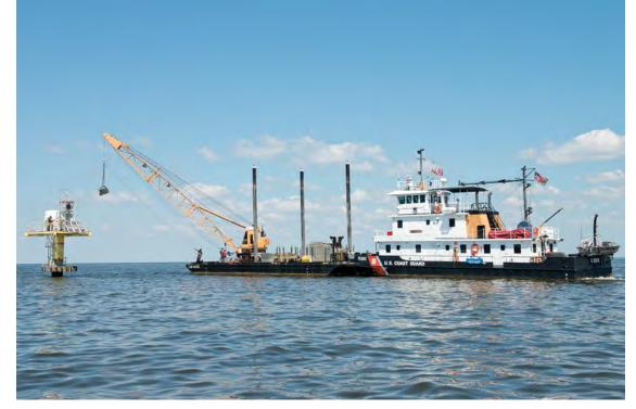
Crewmembers aboard Coast Guard cutter Sledge use the ship's crane to lower a new transformer down to Craighill Entrance front range light Aug. 25, 2014. Crew members from Aids to Navigation Team Baltimore help guide the transformer onto the structure by use of the tag line. © U.S. COAST GUARD PHOTO BY PETTY OFFICER 3RD CLASS JASMINE MIESZALA
