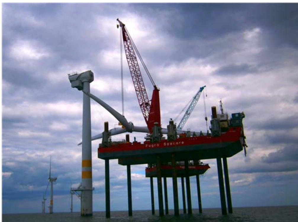
**Figure 3.2. Example of jack-up platforms (Fugro Excalibur and Deep Diver)**
