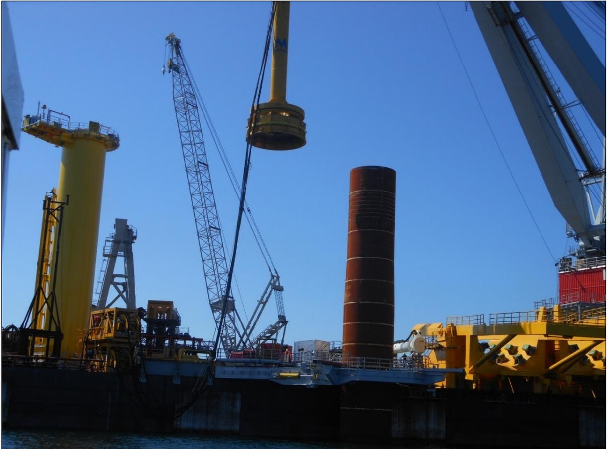
**Figure 4.1: Hammer piling of a monopile**
