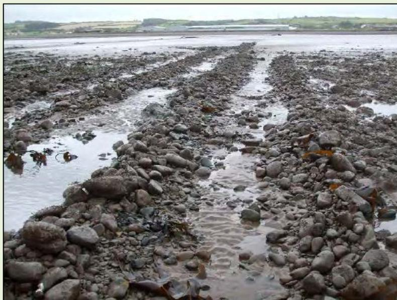
**Figure 5.4: Physical impacts of export cable installation on the lower shore at Robin Rigg Offshore Wind Farm**
