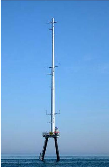
**Figure 3-1 Example of Monopole Mast Meteorological Tower with a Tripod Foundation**
