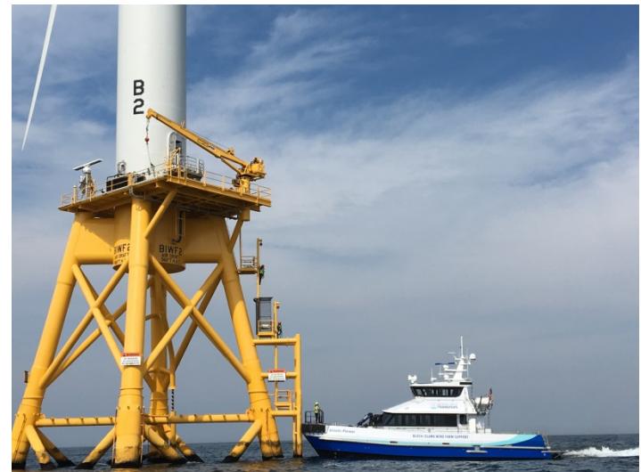
Block Island Wind Turbine with Maintenance Boat
