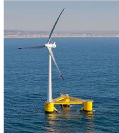
**A full-scale prototype of the WindFloat device**
