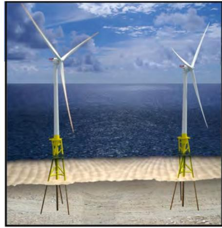
*Beneath the surface: This graphic illustrates the proposed foundations for the two VOWTAP turbines. Specific foundation types for the commercial project have not yet been identified.*
