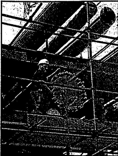
A weldless mechanical MORGRIP pressure test cap fitted to a pipe end ready for hydrotesting the line system. The integrity of the MORGRIP seal having been established by external testing before flooding the line.
