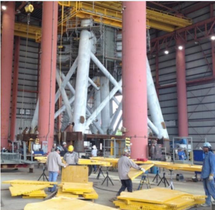
Workers at Gulf Island Fabrication built the steel jackets and decks for the first American offshore wind project.
