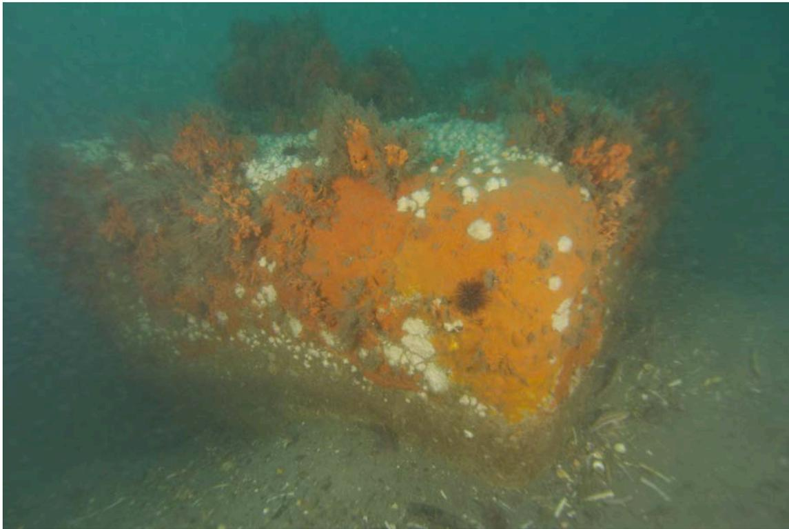
**Figure 5. Target CR002 was determined by BOEM to be a concrete buoy mooring anchor and will not be considered further in this Finding.**
