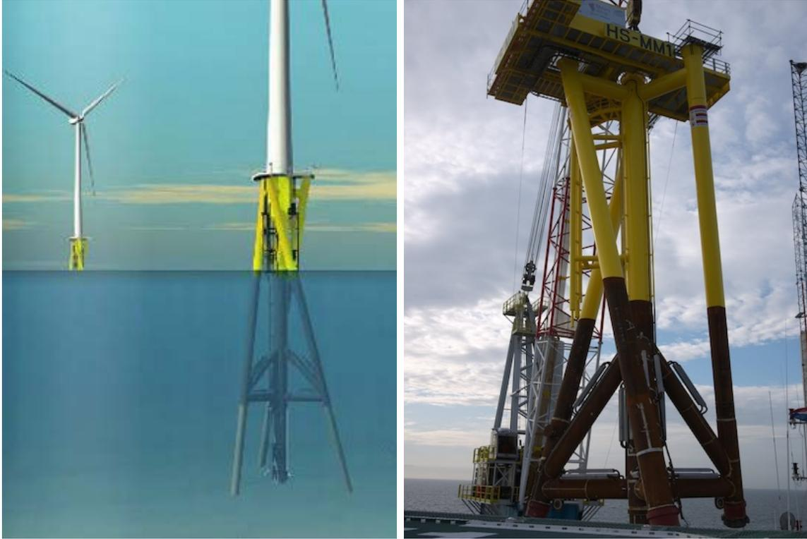
**Figure 2. Inward Battered Guide Structure (IBGS) or "twisted jacket" foundation support structure for wind turbines. Left: Keystone Engineering. Right: National Renewable Energy Laboratory**
