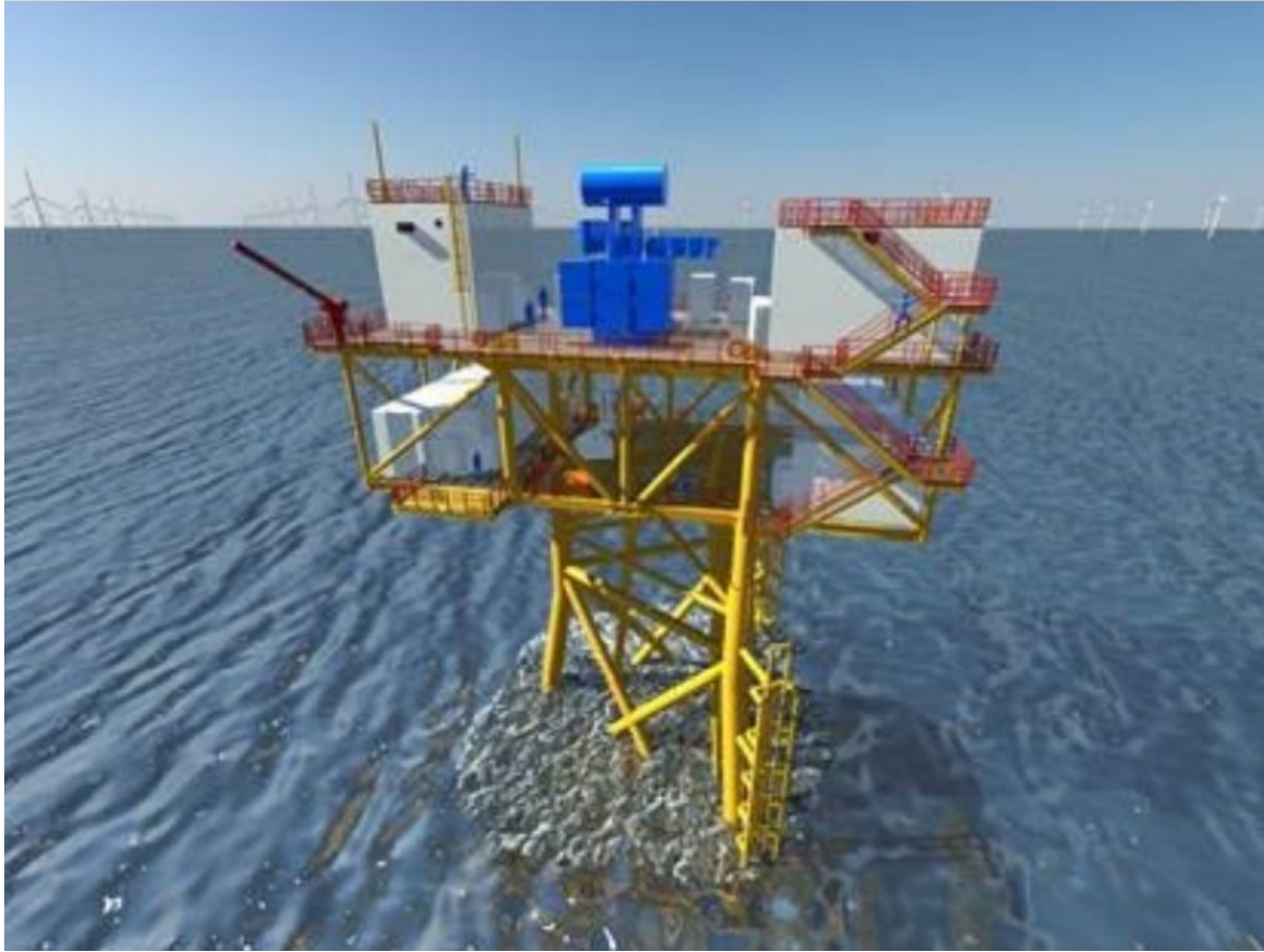
Figure 3-6. Conceptual design for the OSS installed on a jacket foundation
