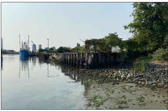
Photograph 3. Overview of partially collapsed wood and concrete bulkhead facing the marina. View to the south.
