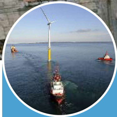
Navigation Channel and Wet Storage
