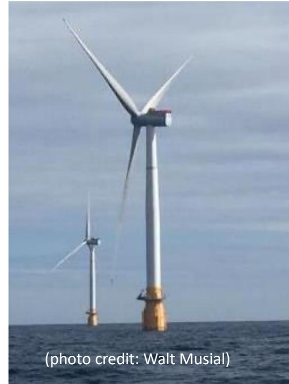
**Five Siemens 6.0-MW Wind Turbines**
