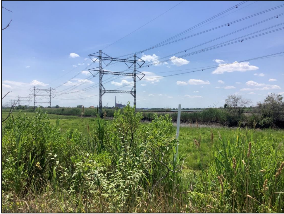
Photograph 1. Standing on River Road looking southwest at W029 (EEM).
