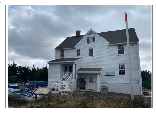
**Description:** The Forked River Coast Guard Station No. 112 is a two-and-one-half-story frame building constructed ca.1932. The building has a cross-gable roof, and clapboard siding, and rests upon a high basement. Currently used as a nature center for Island Beach State Park, the station was determined individually NRHP-eligible by the NJHPO in 1996. The station has also been identified as a contributing resource to the NRHP-eligible Island Beach State Park Historic District.
