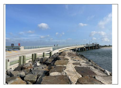
**Description:** The Townsend Inlet Bridge was one of four trunnion bascule bridges designed by Ash Howard Needles & Tammen and erected in Cape May County between 1938 and 1940. Moveable bridges were necessary to facilitate vehicular traffic between the barrier island resorts while still allowing boat traffic to navigate the inlet's confluence with the Atlantic Ocean.
