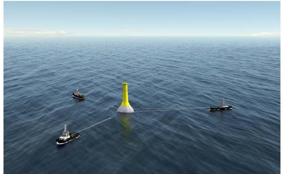
Gravity Foundation Transport via Tugboats
