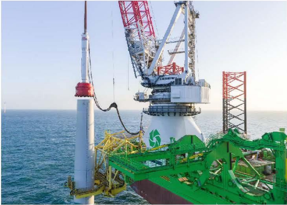
Pile Driving of a Monopile
