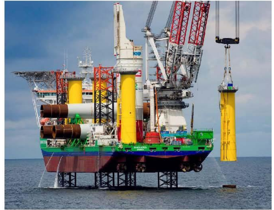
Transition Piece Installation from a Jack-Up Vessel
