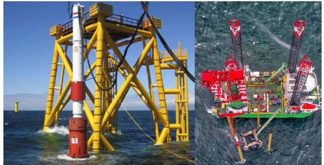
Pile Driving of a Jacket Pile
