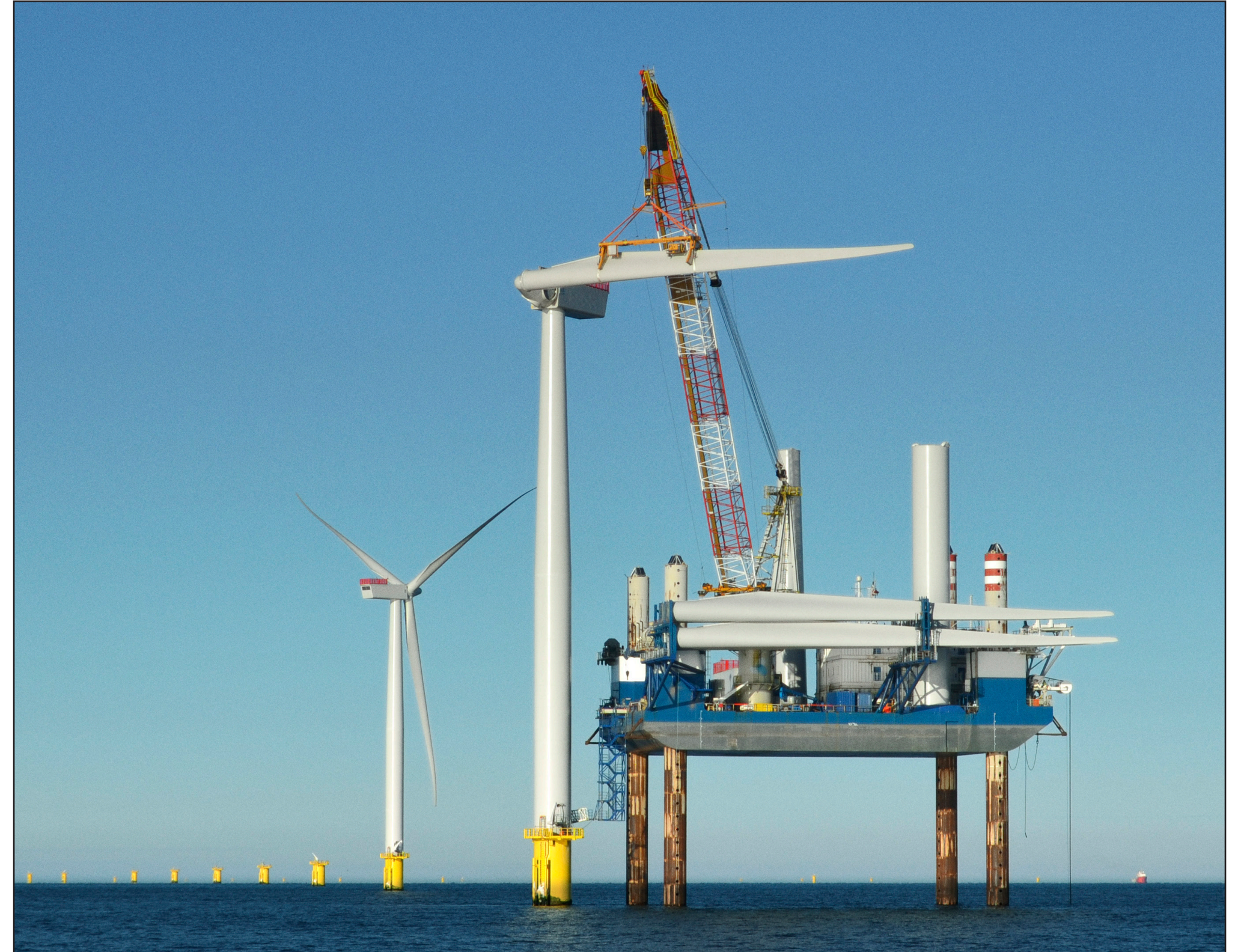
Wind Turbine Installation
