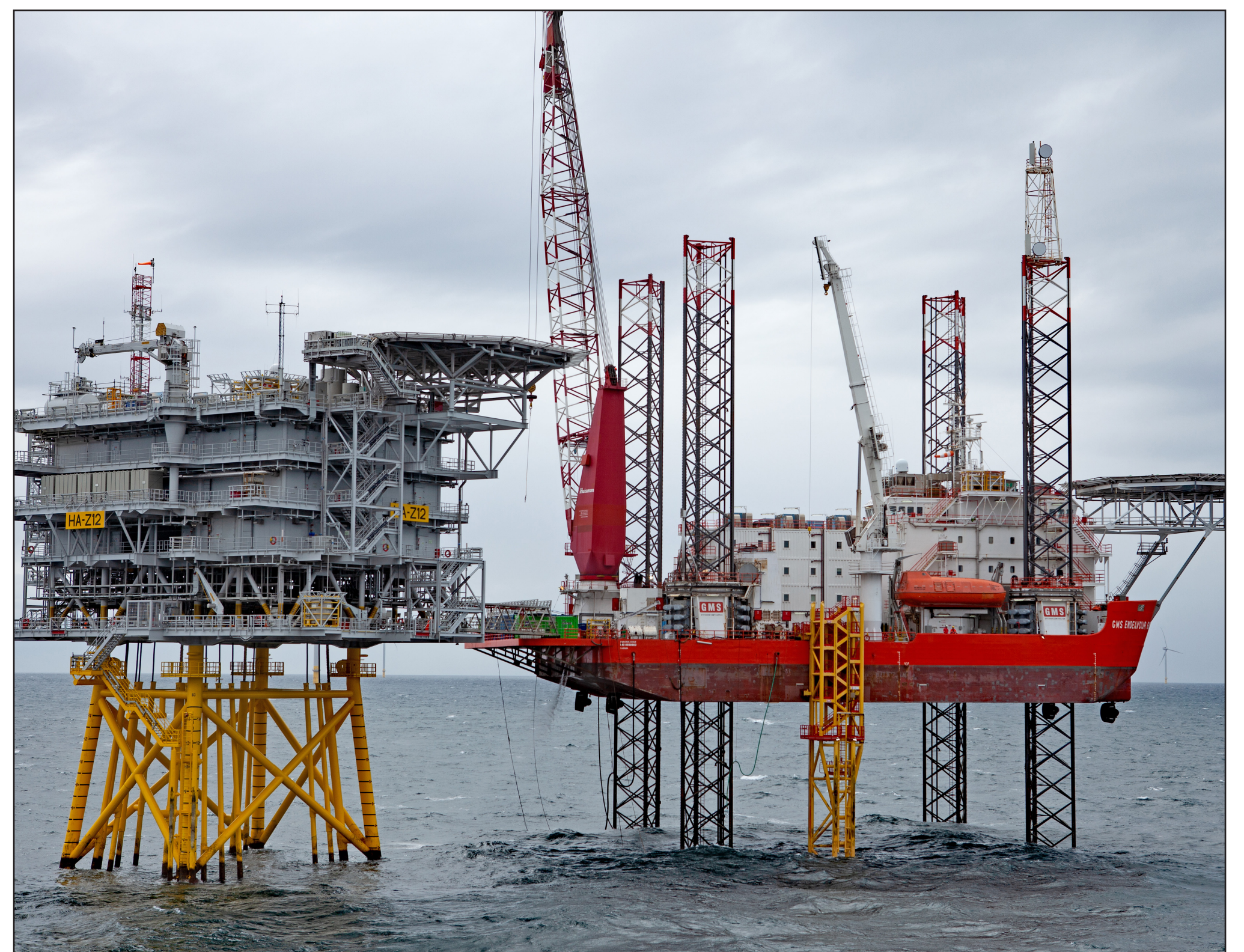
Installation of Offshore Substation
