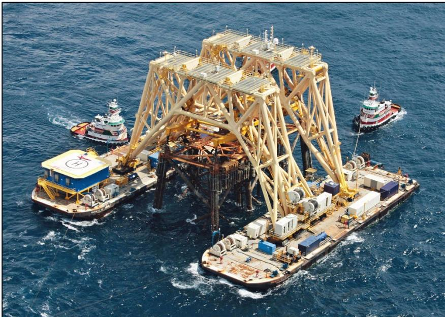
**FIGURE A-2 Versabar bottom feeder lift system (Source: Versabar, Inc. 2017)**
