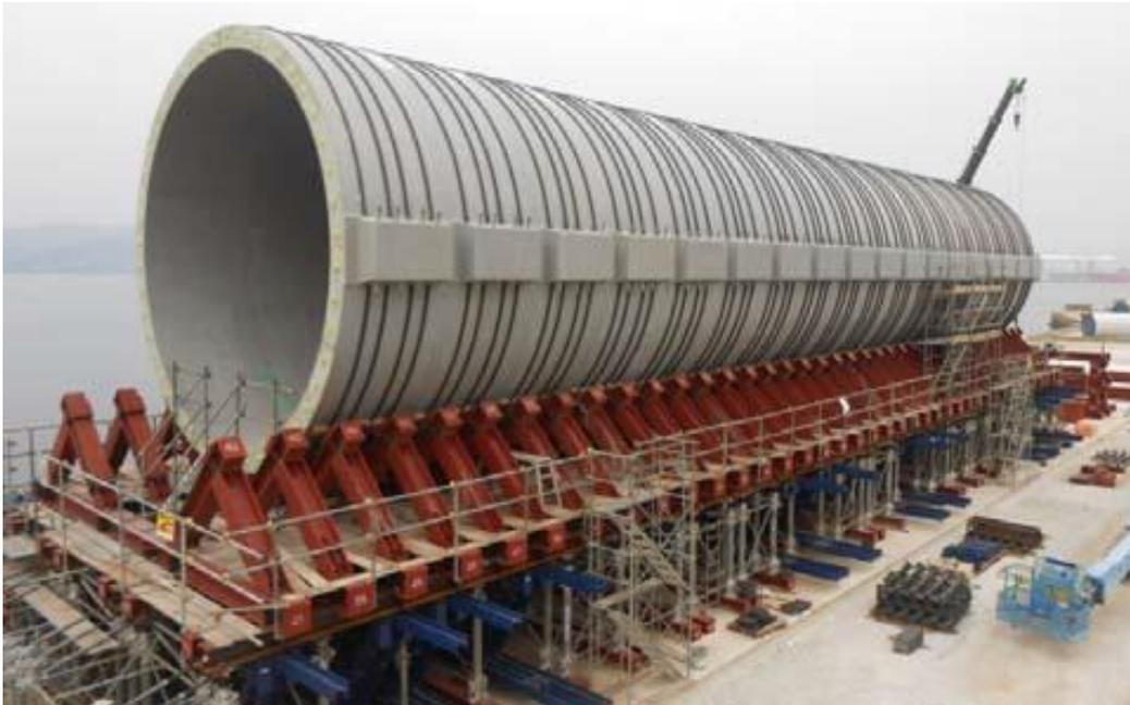
**Figure 47 Concrete Part of the Hybrid Spar – Sakiyama Project**
