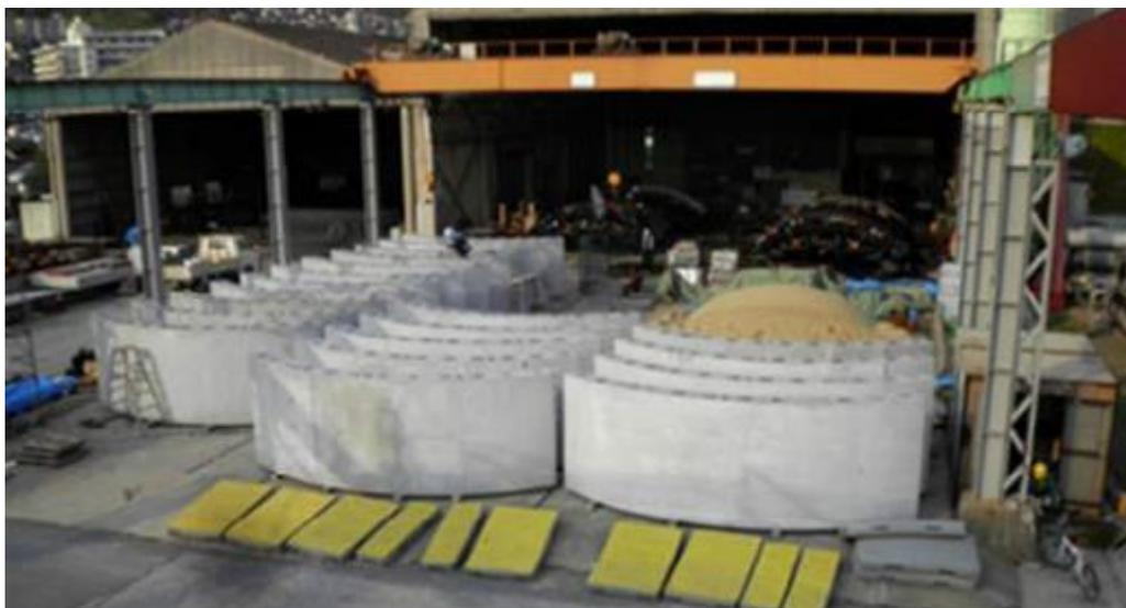
Figure 46 Fabrication of Concrete Segments – Sakiyama Project
