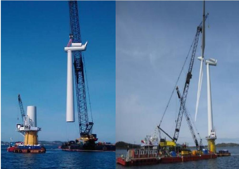
**Figure 52 Hywind Demo – Inshore Assembly of a FOWT (Stateoil, 2009)**
