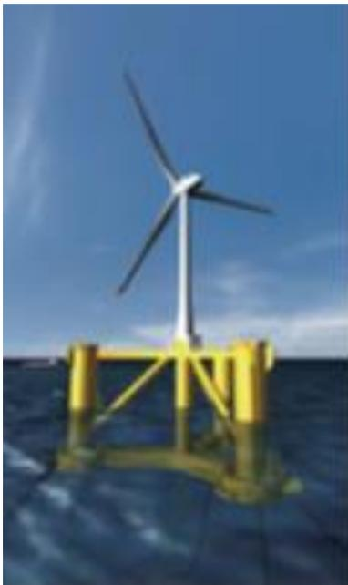
The compact semi-submersible (Fukushima Mira) was designed by Mitsui Engineering & Shipbuilding Co., Ltd. (MES). This floater consists of one center column supporting the wind turbine, three side columns, three braces, main deck beams, and pontoon beams.
