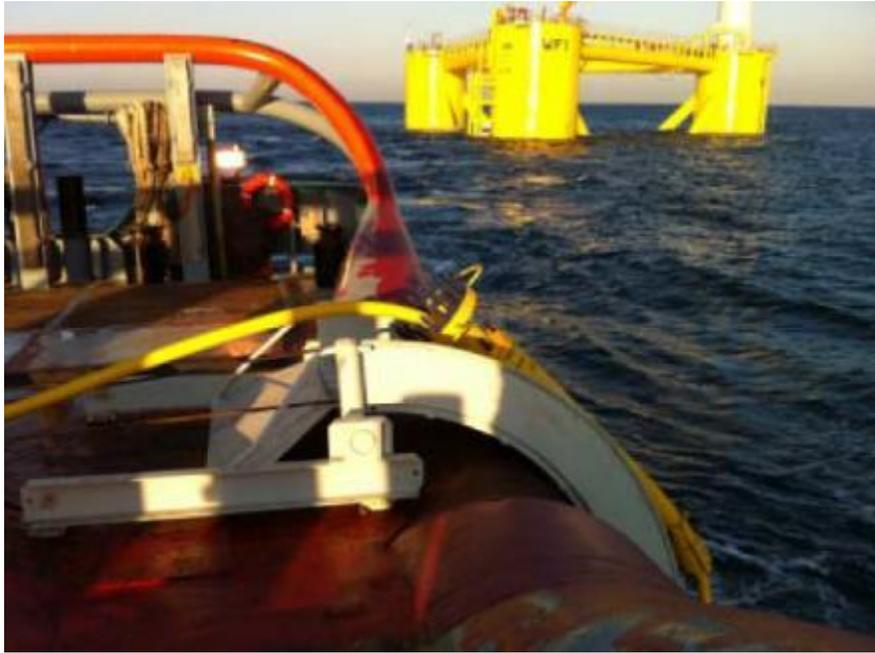
**Figure 55 WindFloat 1 (WF1) – Bend Stiffener of the Power Cable over the Vessel Stern (Cermelli, Roddier, and Weinstein, 2012)**
