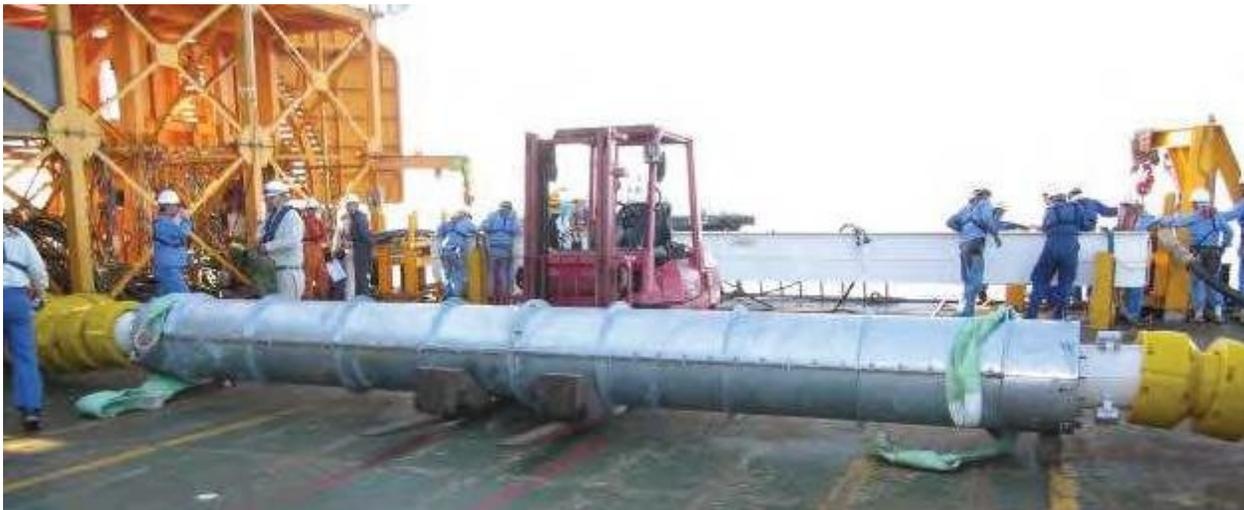
Figure 38 Fukushima FORWARD Project 66 kV Transition Joint (Fujii and Tanaka, 2013)
