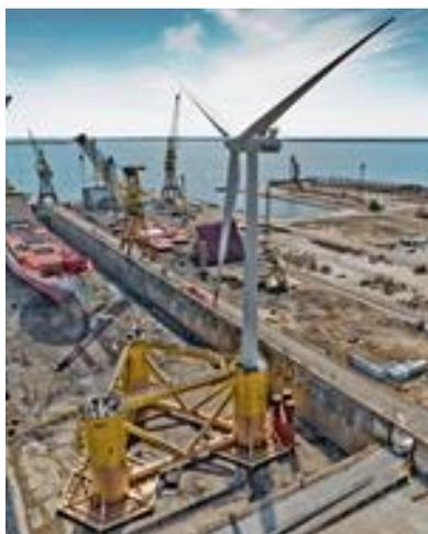
Figure A-2 The 2MW WindFloat 1 (WF1)
