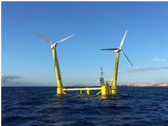
**Figure A- 10 The W2Power 1:6 prototype**
