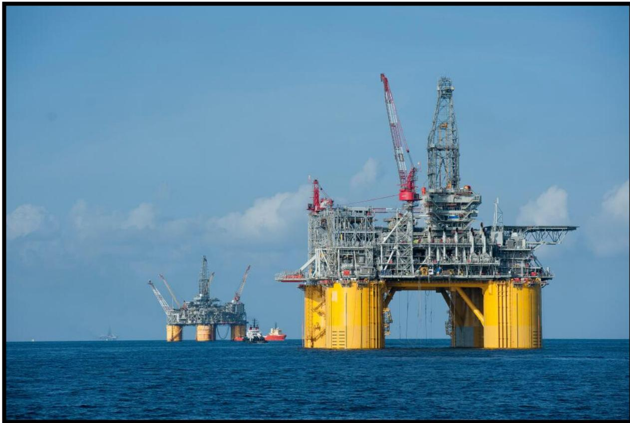
Cover: Shell's Olympus tension leg platform (TLP) is part of the Mars B development (forefront), located in 3,100 feet of water (945 m), installed in 2013 and designed with a production capacity to exceed over 100,000 BOE per day. Other owners include BP. Photo from Offshore magazine (accessed on 10/25/2017): <http://www.offshore-mag.com/articles/2013/08/shell-s-olympus-tlp-in-place-on-target-for-2014-startup.html>
