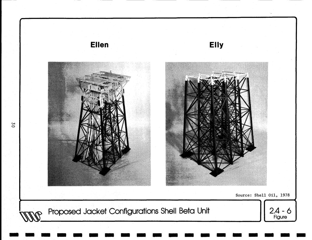
an earthquake environment. The platforms have been designed by Shell for a two-level design requirement as outlined in API RP 2A. For the first-level earthquake criteria, Shell's design specification is that the platforms resist shaking, without damage. In this case, they have selected a peak horizontal acceleration of 0.25 g. Shell's analysis is that the probability that the platform locations will experience this earthquake activity is about 0.005 per year - a 200year recurrence interval.
