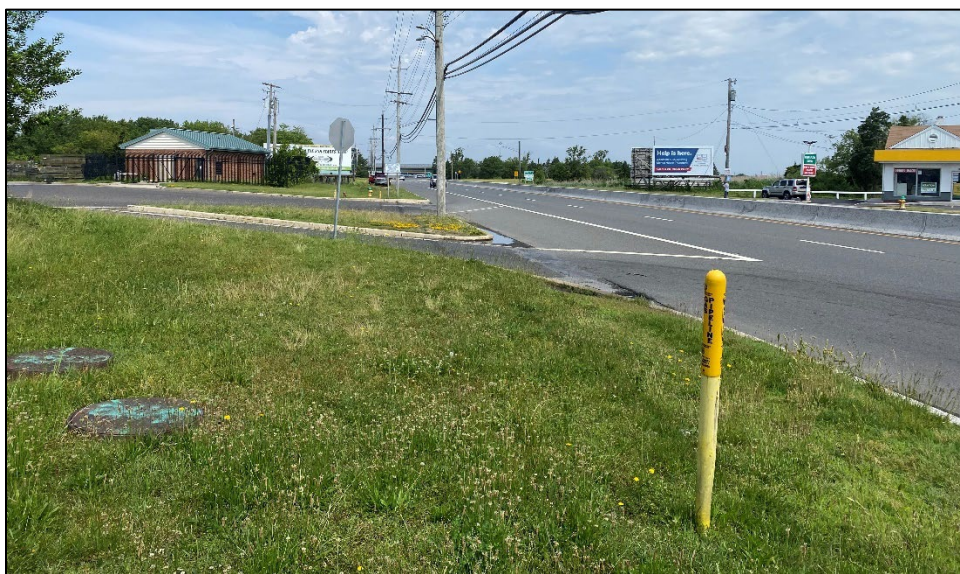
Photograph 40. Overview of Cardiff Onshore Route option along U.S. Route 40. Note the multiple buried utilities adjacent to the road. View to the northwest.
