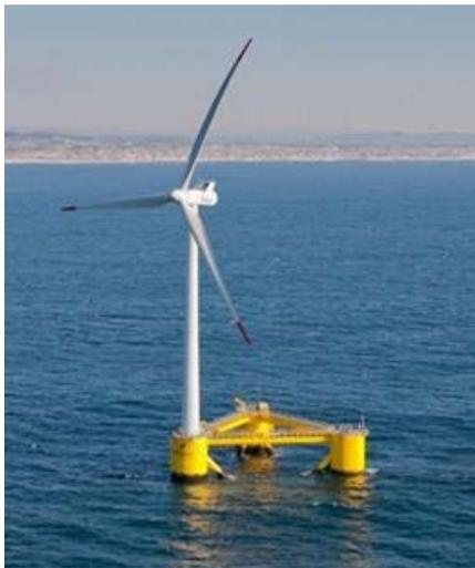
**A full-scale prototype of the WindFloat device**
