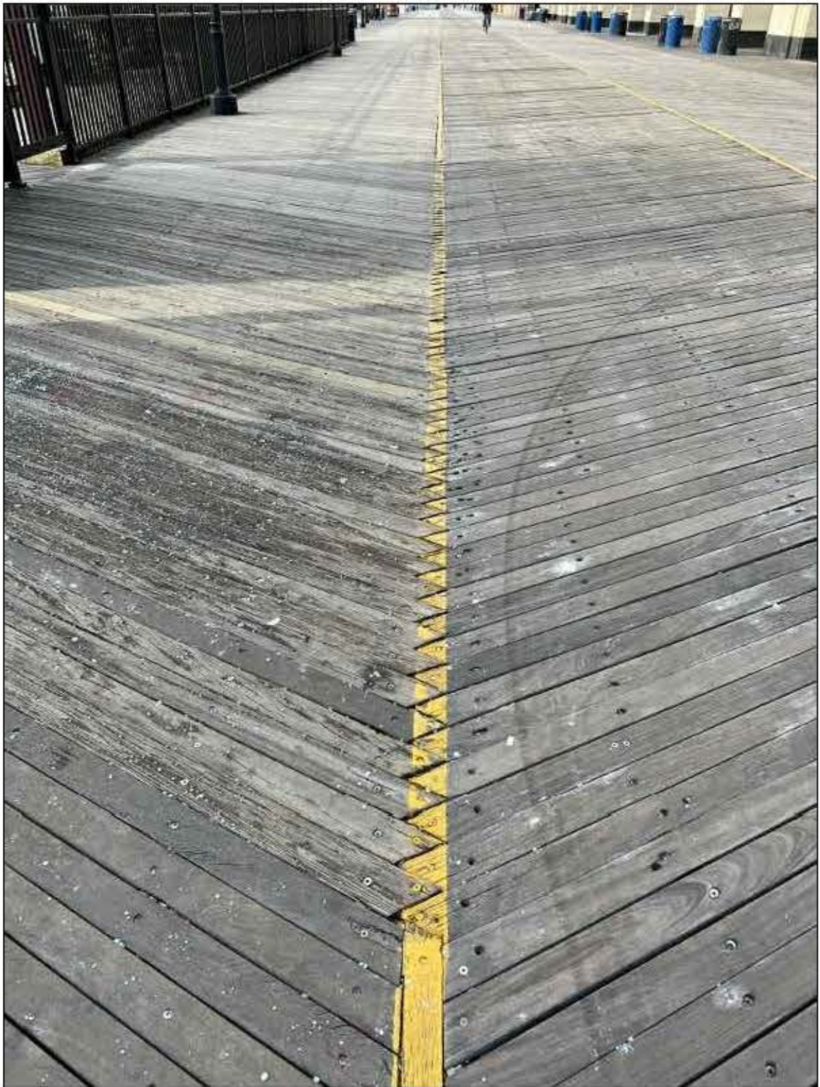
EXISTING "HERRINGBONE" PATTERN DECKING TO BE REMOVED AND INSTALL NEW "RIBBON" BOARD & JOIST
