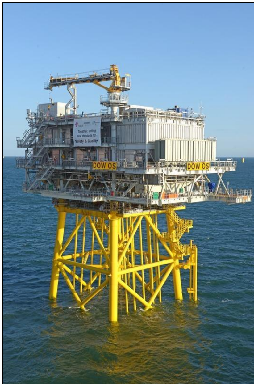
Figure AA-5 Example of an Offshore Substation on a Suction Bucket Jacket Foundation (Equinor-Operated Dudgeon Offshore Wind Farm)
