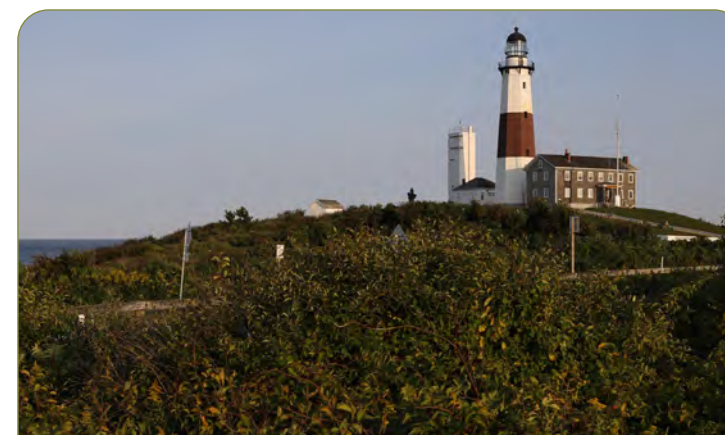
Context Photo: View to the Southeast
