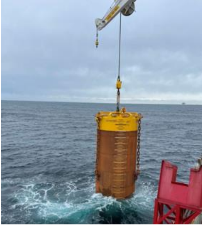
Figure 3-1. Representative Photograph of a Suction Bucket
