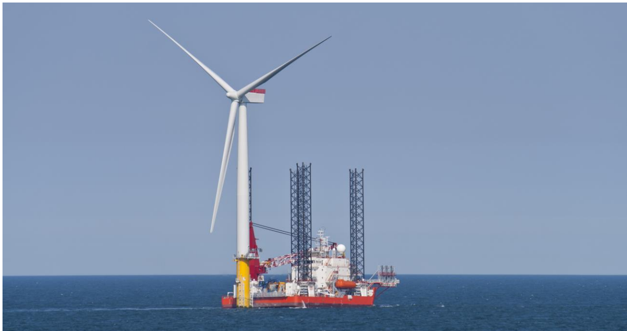
FIGURE 3-15. EXAMPLE OF A JACK-UP VESSEL INSTALLING A WTG
