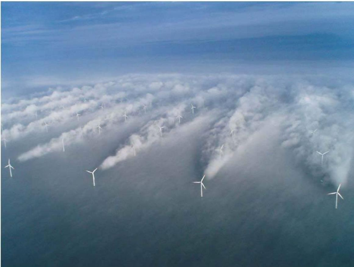
**Figure 1. Horns Rev 1 Visible Fog Wake**
