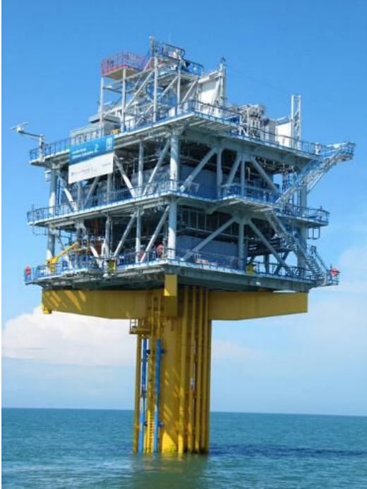
Figure 6.1.1-5 - Indicative monopile foundation offshore substation (London Array).
