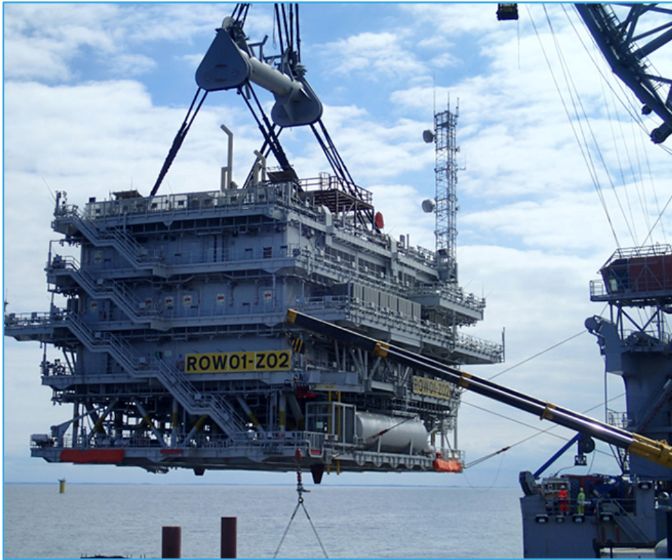
Figure 6.1.2-12 - Installation of an offshore substation.
