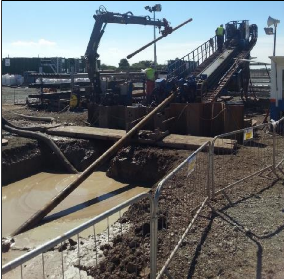
Figure 6.2.2-2 - Example HDD rig in operation at entry point.
