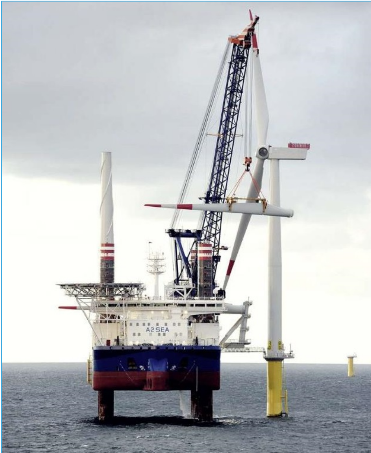
Figure 6.1.2-10 - Installation of a WTG blade.
