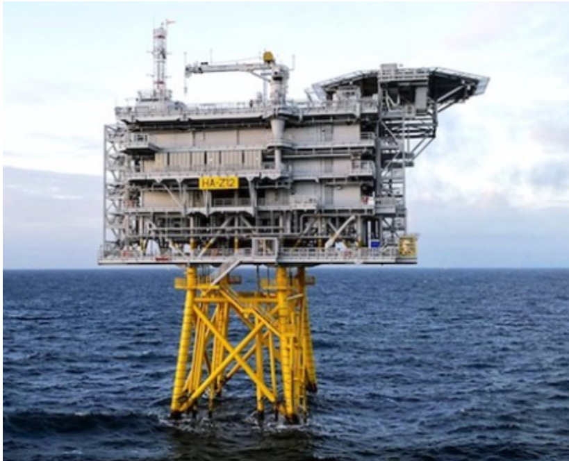
Figure 6.1.1-7 - Indicative offshore substation with helideck (Hornsea I).
