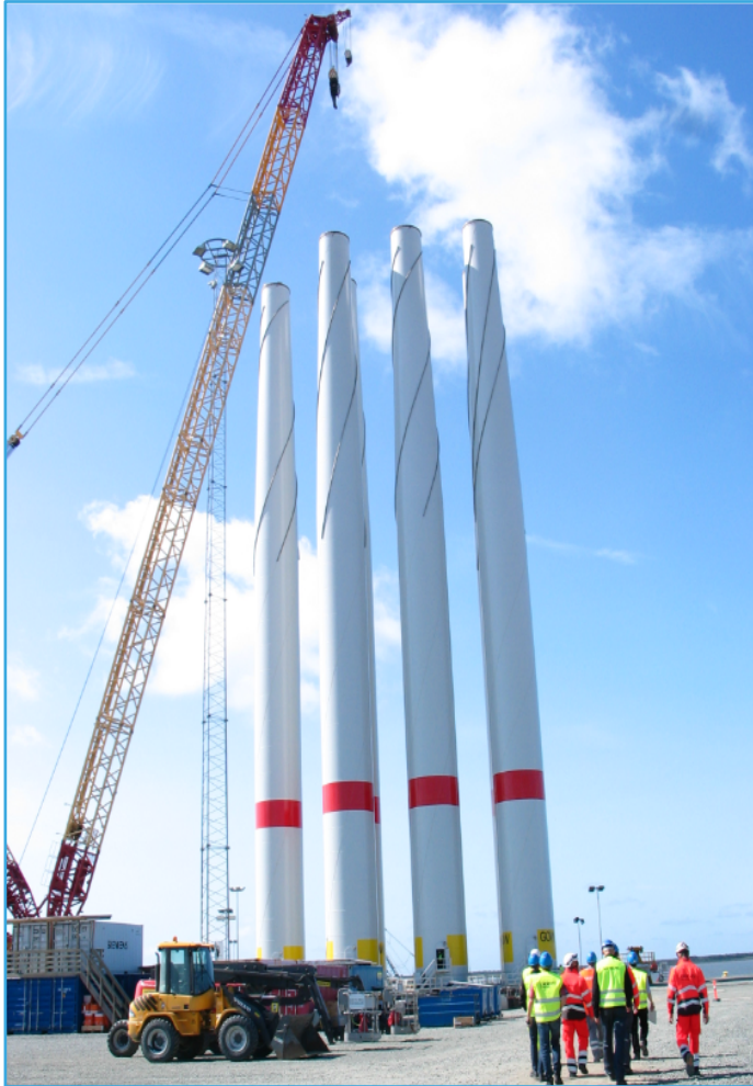
Figure 6.1.2-6 - Towers assembled and ready for load-out.
