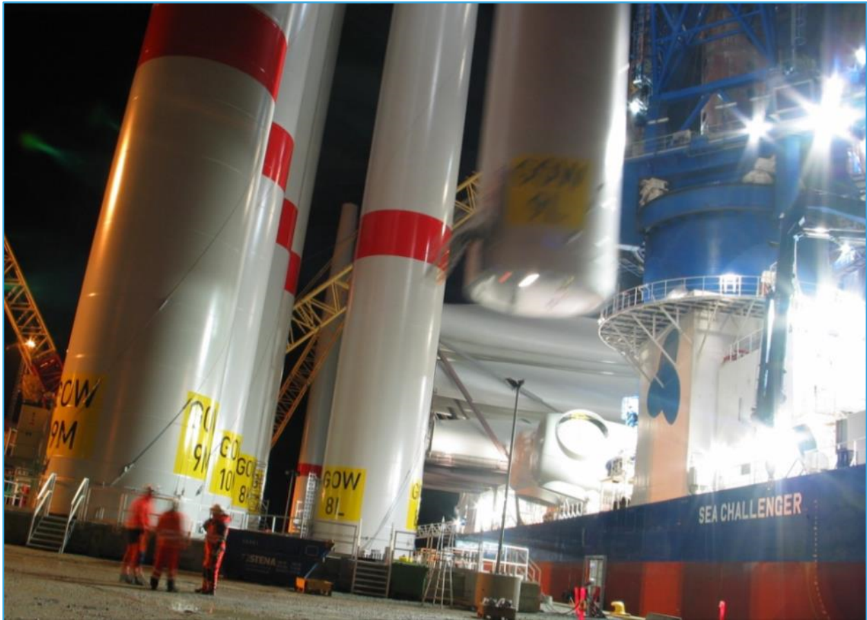
Figure 6.1.2-9 - Loading towers onto installation vessel.
