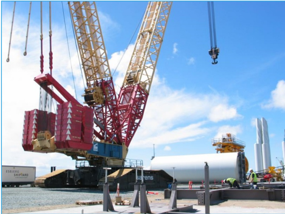
Figure 6.1.2-4 - Upending of tower section in load-out port.
