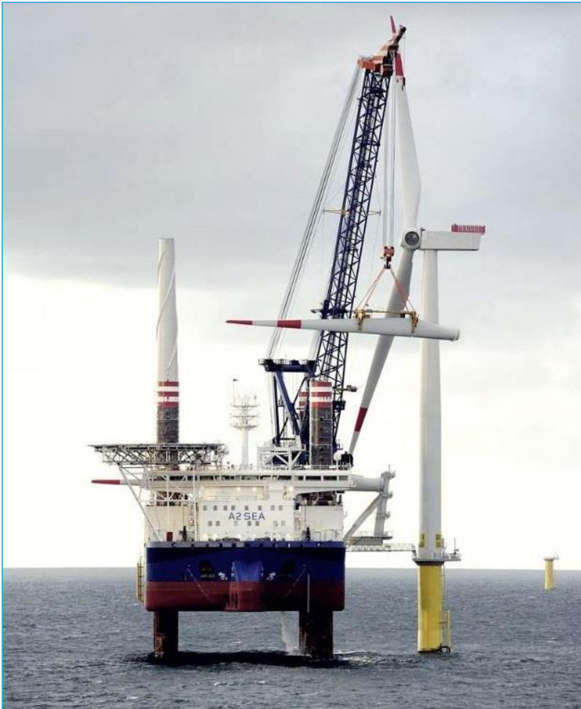
Figure 6.1.2-10. Installation of a WTG blade.
