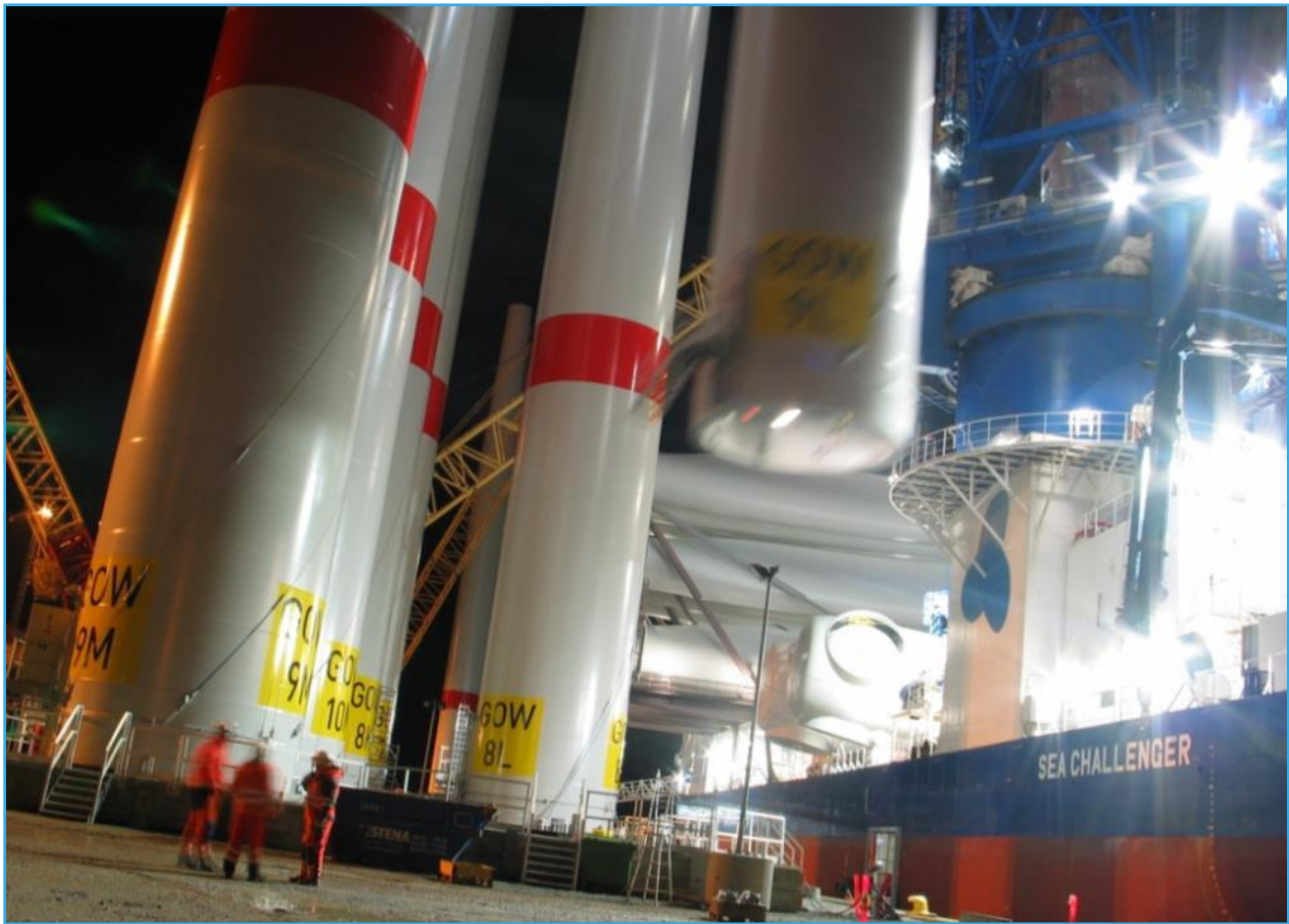
Figure 6.1.2-9. Loading towers onto installation vessel.
