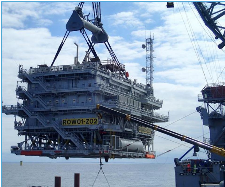
Figure 6.1.2-12. Installation of an offshore substation.
