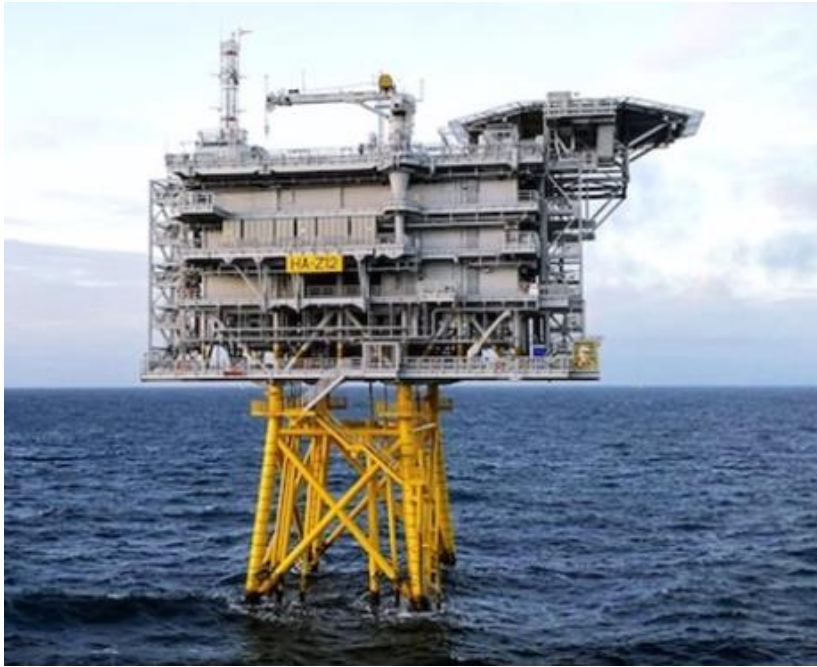
Figure 6.1.1-7. Indicative offshore substation with helideck (Hornsea I).
