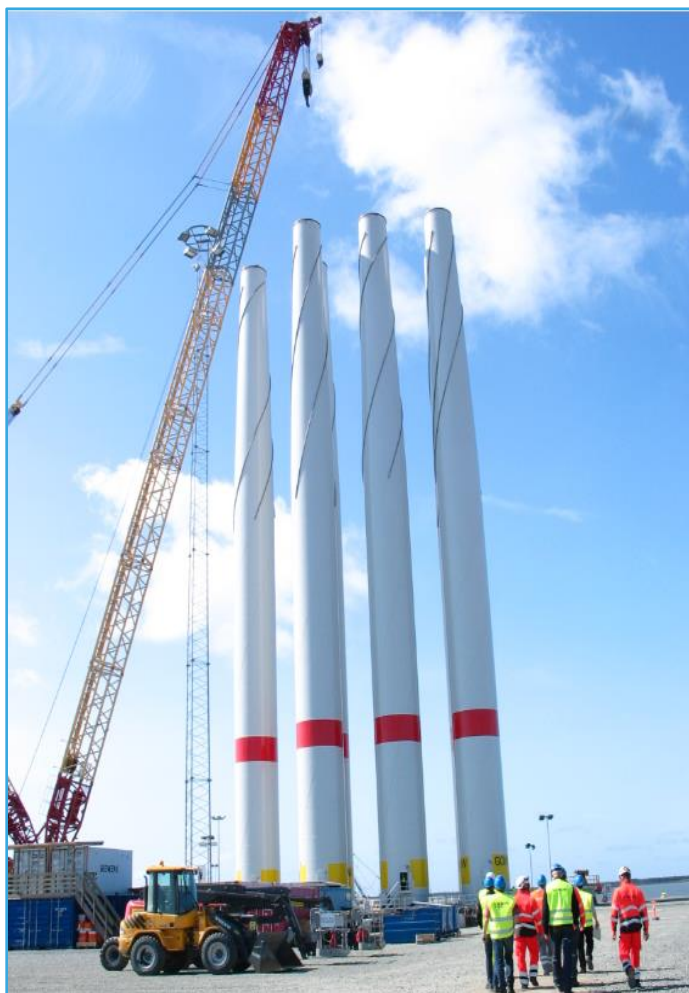
Figure 6.1.2-6. Towers assembled and ready for load-out.
