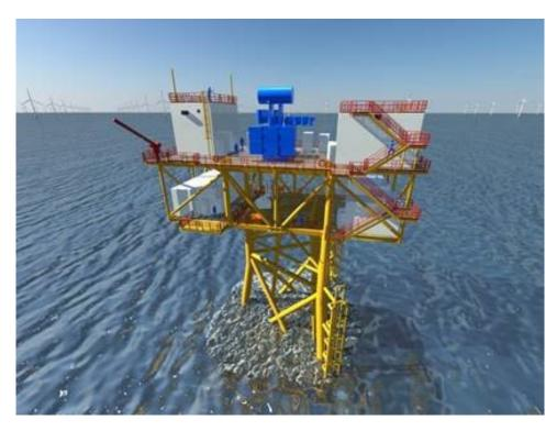
Figure 2-7. OSS on Jacket Foundation Source: HSM Offshore
