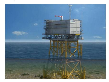
Figure 3-3. Example High-Capacity OSS with Jacket Foundation and Skirt Piles¶ Source: Tennet.eu, Borssele Alpha OSS
