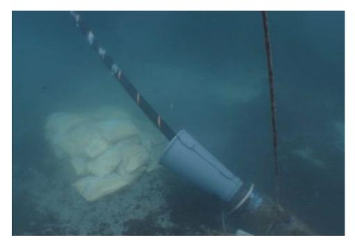
Figure 3-13. Underwater View of Near Shore Cable Pull into HDD Duct¶Source: Nexans.com
