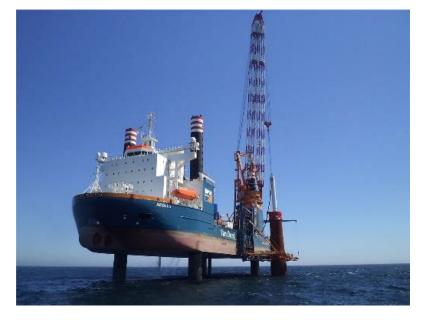
Figure 3-2. Monopile Installation Source: Globalenergyworld.com
