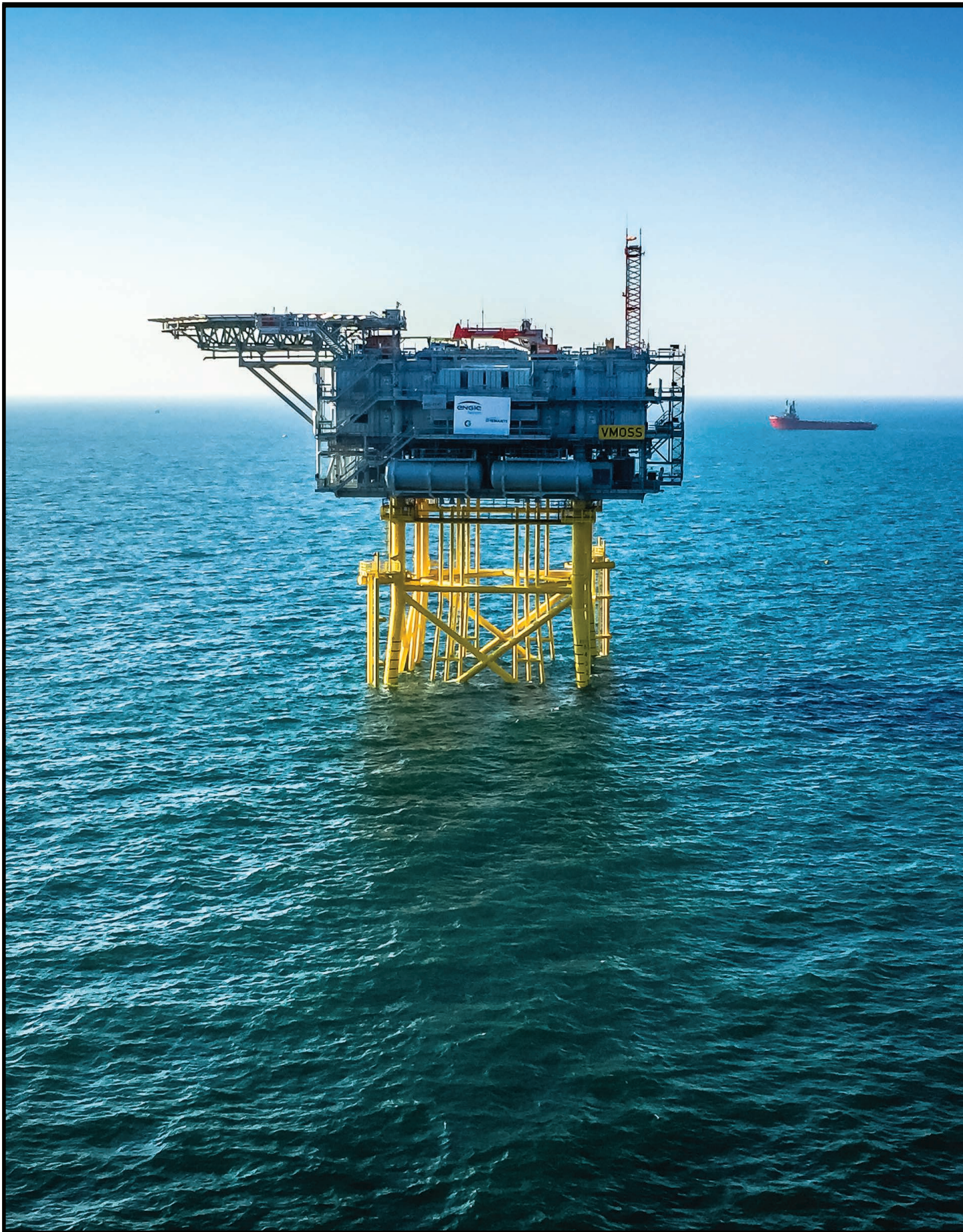
Figure 3 Representative ESP/Booster Station
